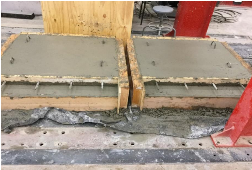
Figure 13: Side-by-side slabs after finishing applied
