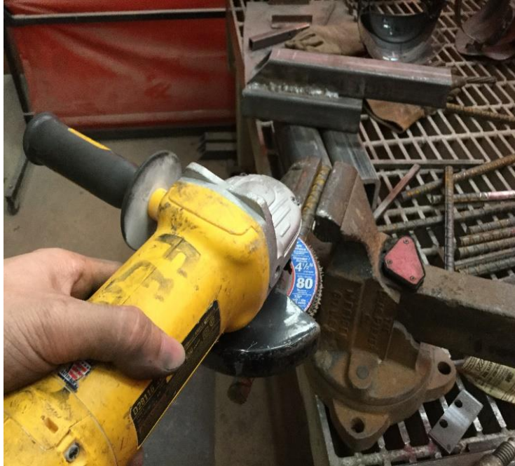
Figure 17: Smoothing splice bar with an angle grinder
