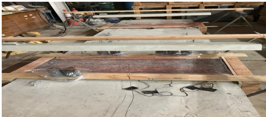
Figure 22: Heat lamp setup to cure UHPC
