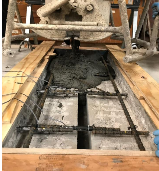
Figure 20: Placement of UHPC connecting two slab panels
