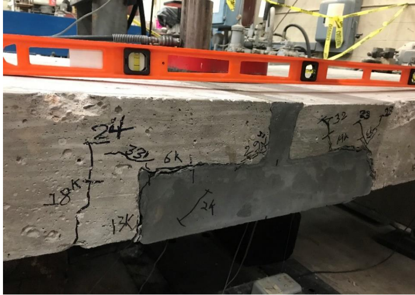
Figure 30: Cracks formed at interface between UHPC and conventional concrete and underneath the load point on the south side
