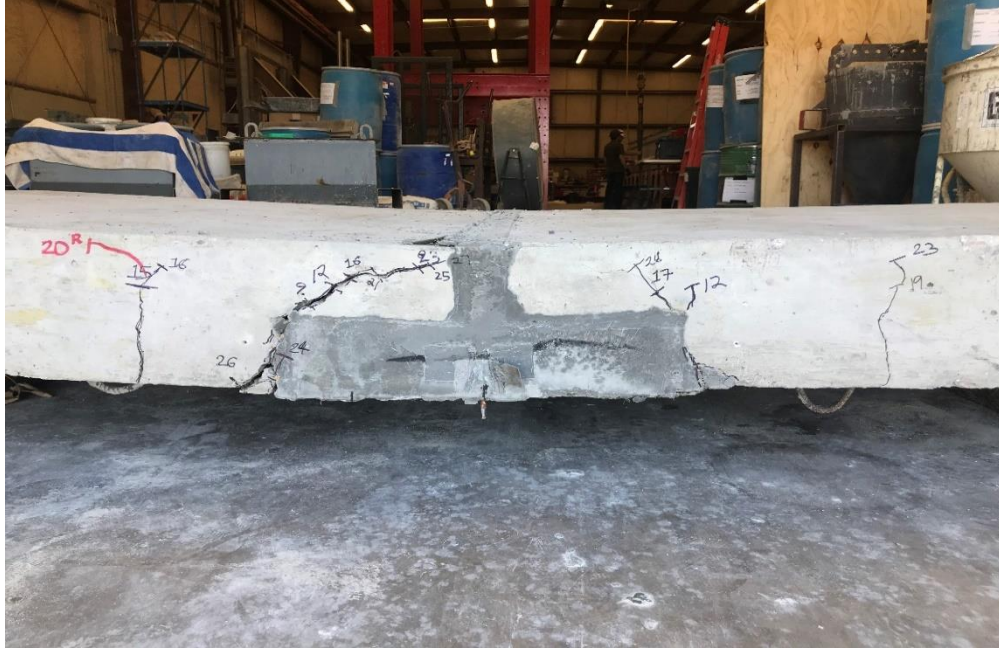
Figure 48: Ductal® slab 1 after part 2 of testing
