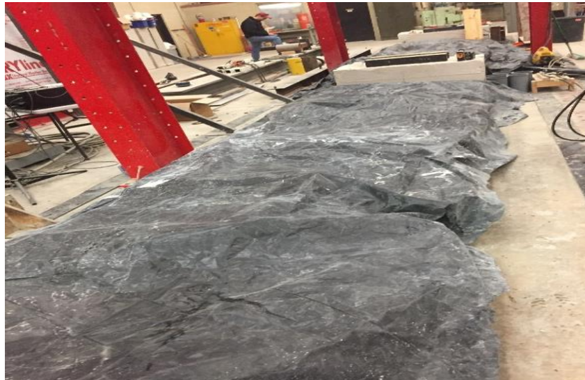
Figure 15: Plastic tarp covering curing concrete panels
