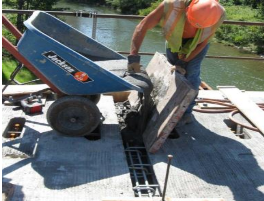
Figure 1: Field-casting and placement of UHPC (Graybeal 2010)
