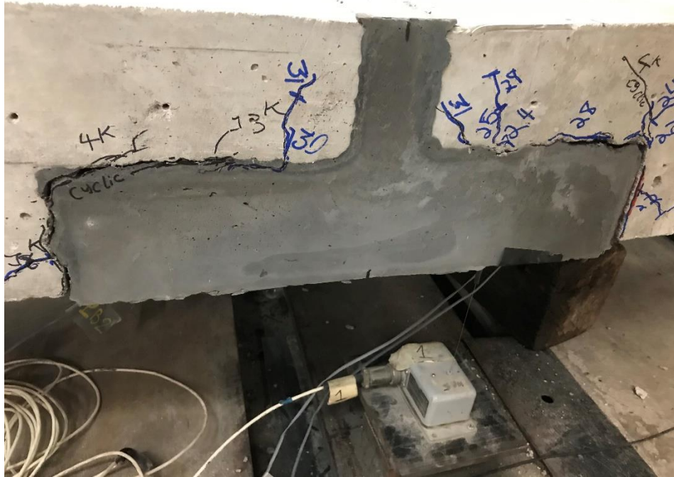
Figure 41: Cracks formed at the conventional concrete to UHPC interface and propagating upward on the south side
