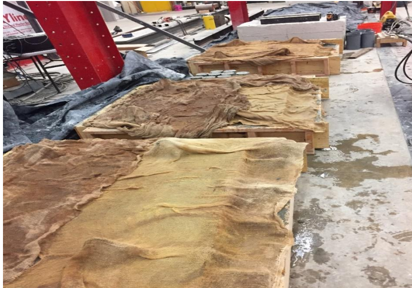
Figure 14: Concrete panels curing covered by wet burlap
