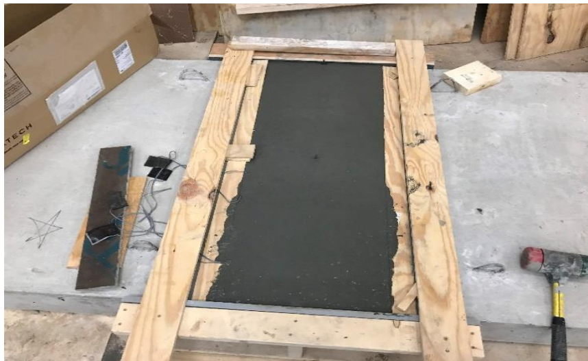
Figure 21: Self-consolidating UHPC filling the joints
