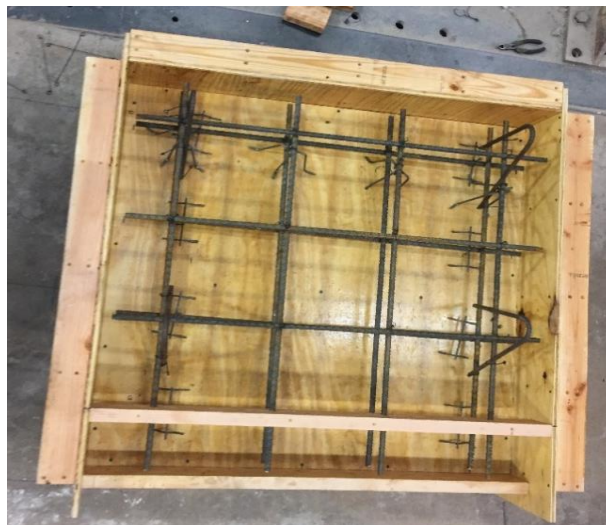
Figure 7: Slab formwork and steel reinforcement
