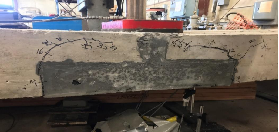
Figure 54: Cracks on the south side of Ductal® slab 2 after part 1 testing
