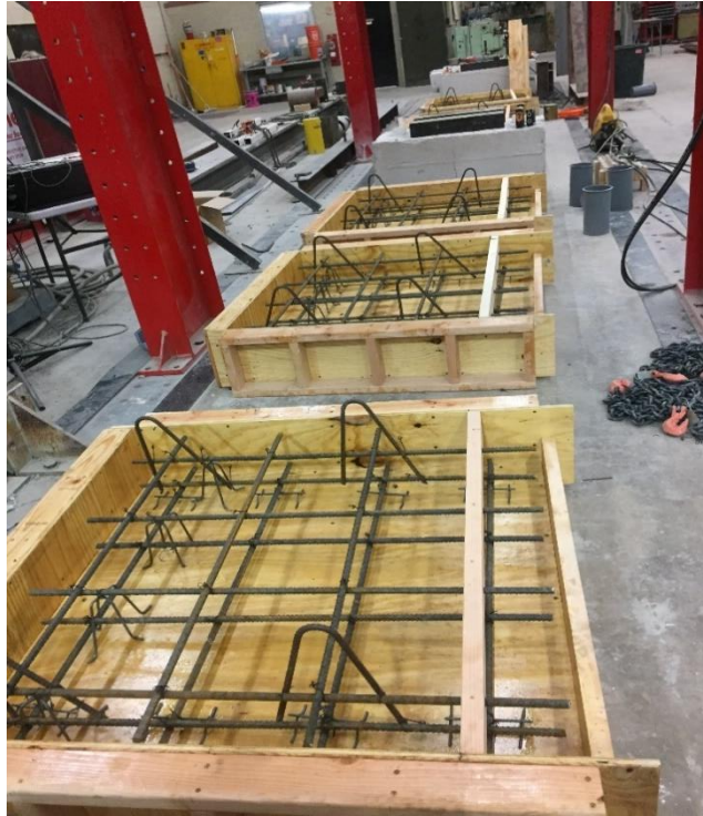
Figure 8: Formwork prepared for concrete casting
