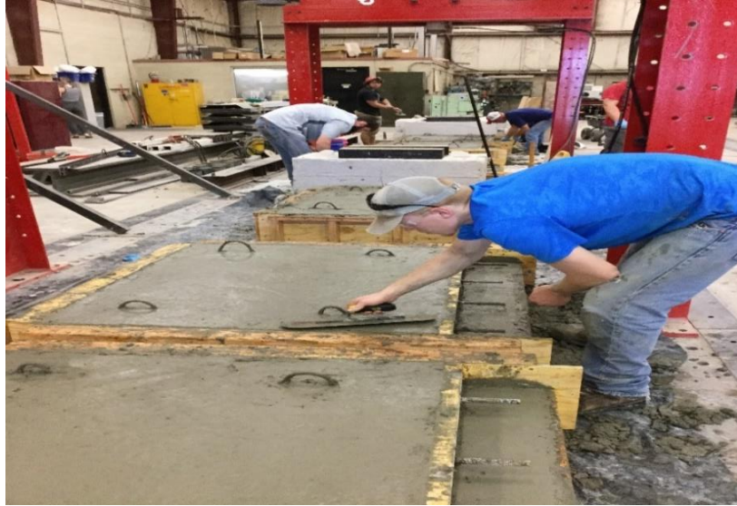
Figure 12: Finishing application on the top surface of the slab
