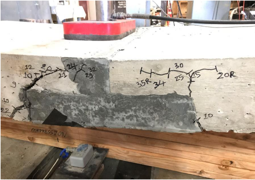
Figure 57: Cracks on the north side of Ductal® slab 2 after part 2 testing
