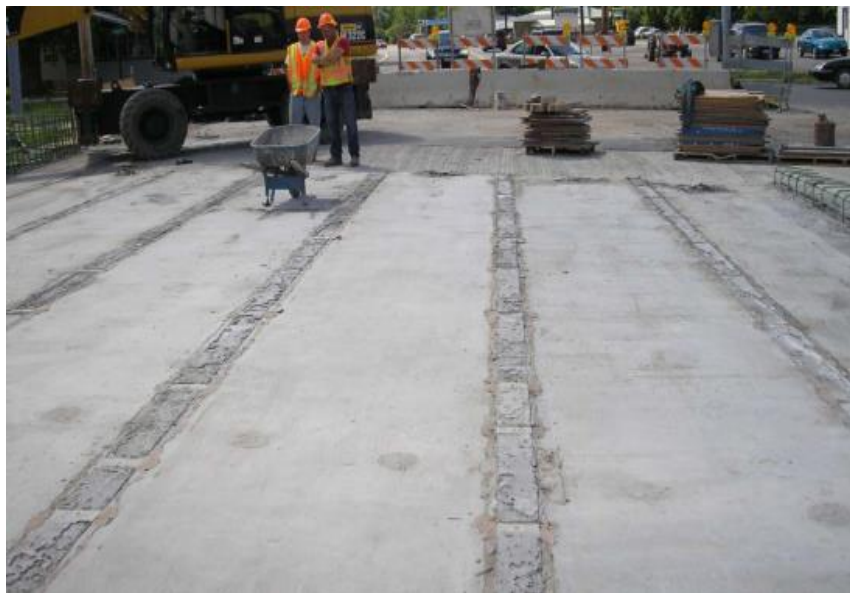
Figure 2: Longitudinal connections using UHPC (Graybeal 2010)
