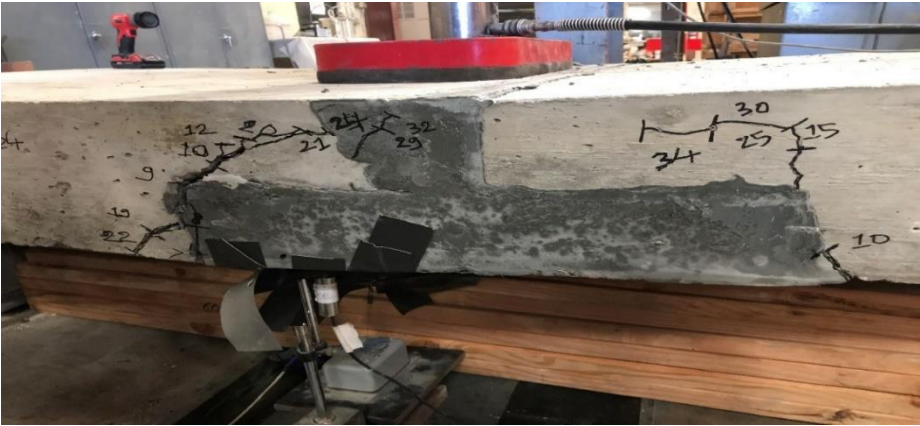
Figure 53: Cracks on the north side of Ductal® slab 2 after part 1 testing
