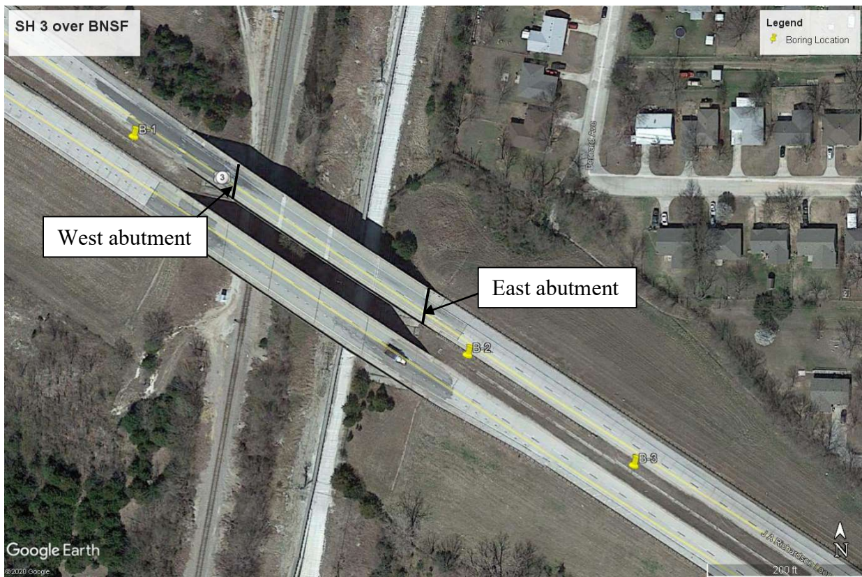
Figure 49. SH 3 over BNSF Boring Locations
