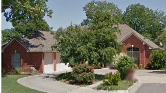
Figure 4.3. Profile of the front of the test home.
