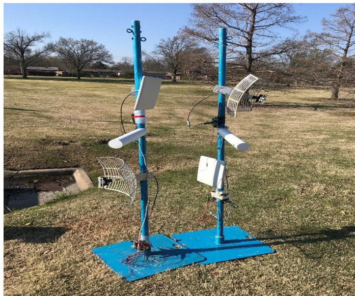
Figure 18. Antenna Setup on the poles used in third test.
