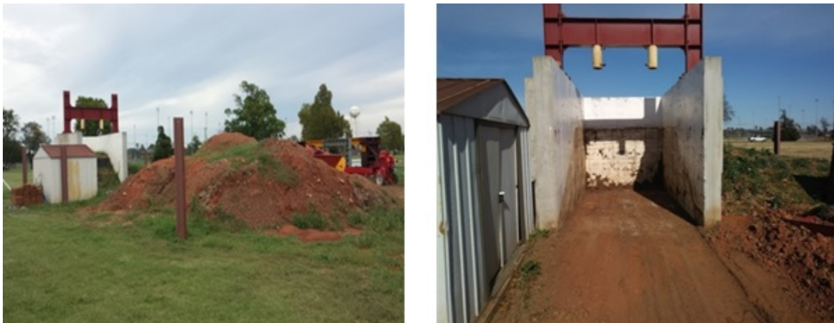
Figure 1. (Left) Condition of the test station at the start of the project; (Right) Test box after cleaning and clearing in Task 1
