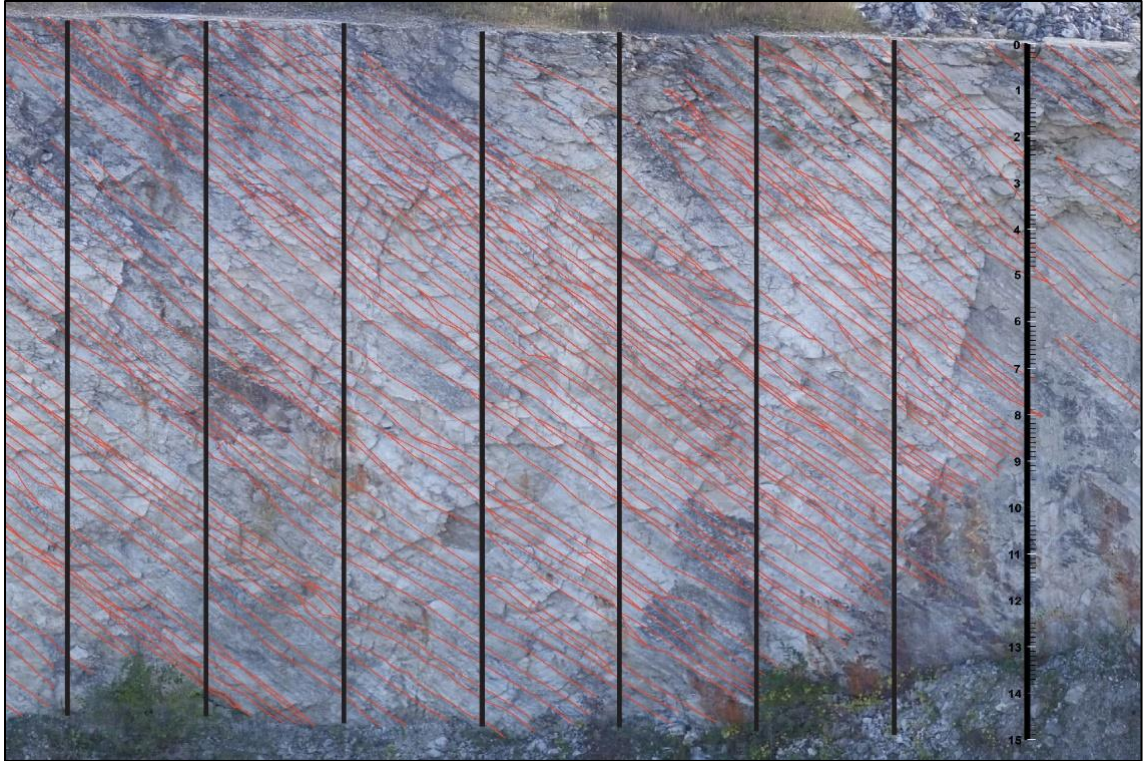
Figure 16: A 21 m section of the southern wall of the Western section showing bed tracings and the pseudowells at 3 m spacing. This was the second step in the process of creating pseudo measured sections. The meter-scale lateral (downslope) variability and the dm- to m-scale vertical variability of the slope beds can be observed in this image. Scale bar is 15 m and is subdivided into meter and decimeter increments.
