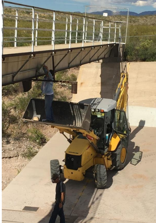
Figure 7: Stream radar mounted on bridge at Walnut Gulch
