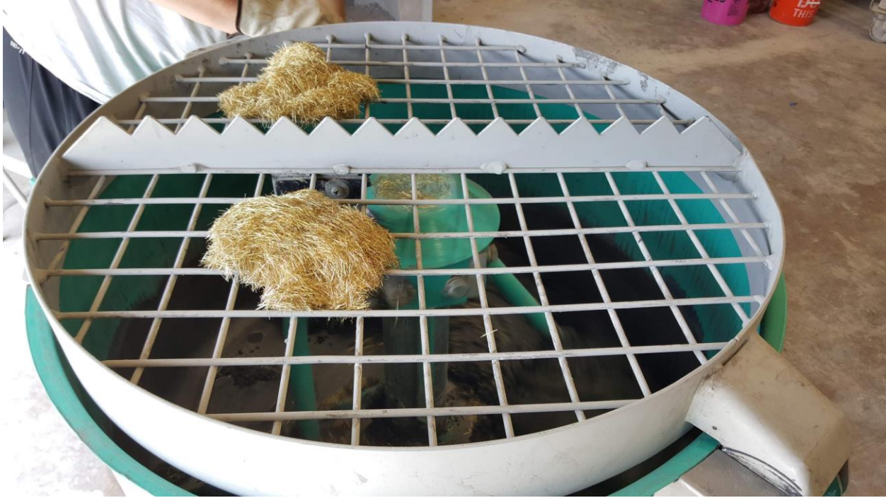
Figure 2: Steel fibers being added during mixing
