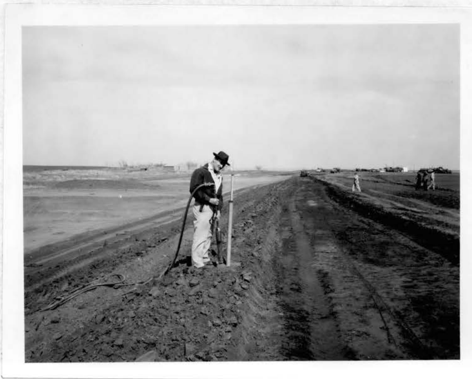
Figure 17. Supplementary compaction of soil around protecting pipe.
