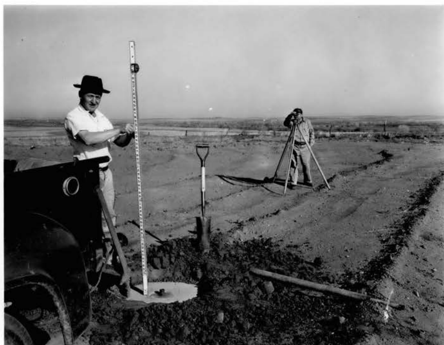
Figure 14. Determining the elevation of the installed plate.
