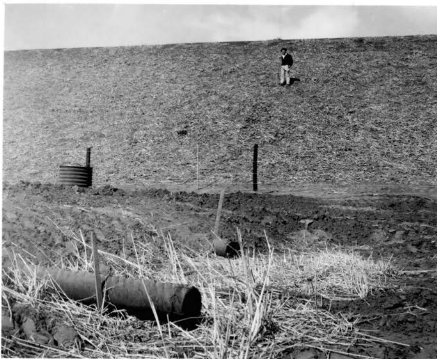
Figure 8. Relative location of Relief Well outfall lines, Relief Well No. 2 and gages in 2:1 slope of Site 16.
