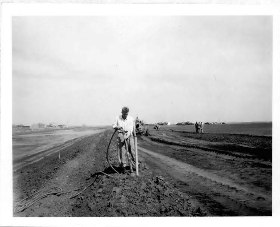
Figure 18. Compacting the soil around the gages using an air-driven tamper.
