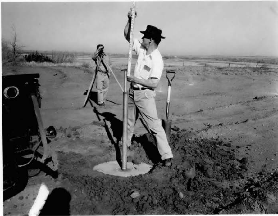
Figure 15. Determining the elevation of the notch in the 1" gage pipe.
