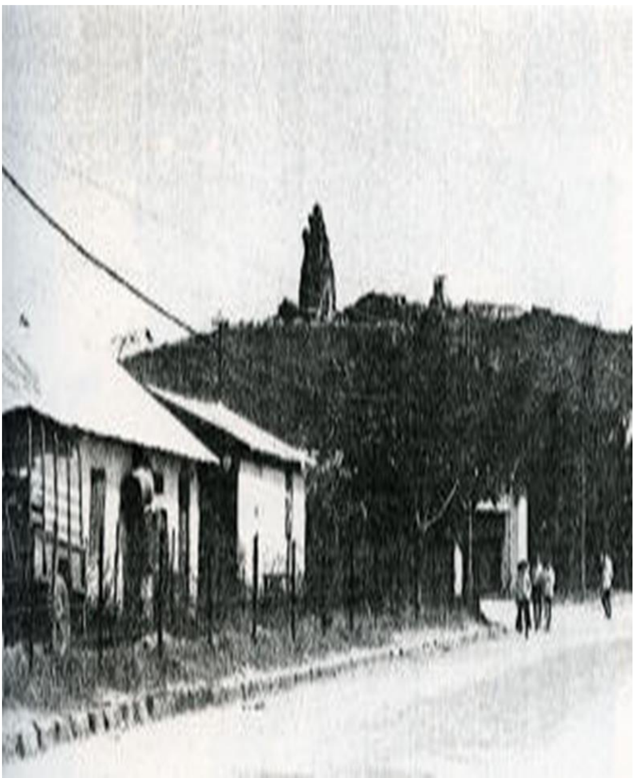
Figure 3.2 Province Interrogation Center
