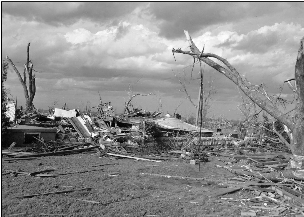
Figure 3: Tornado Damage in Woodward, OK 1947 (NWS n.d.)
