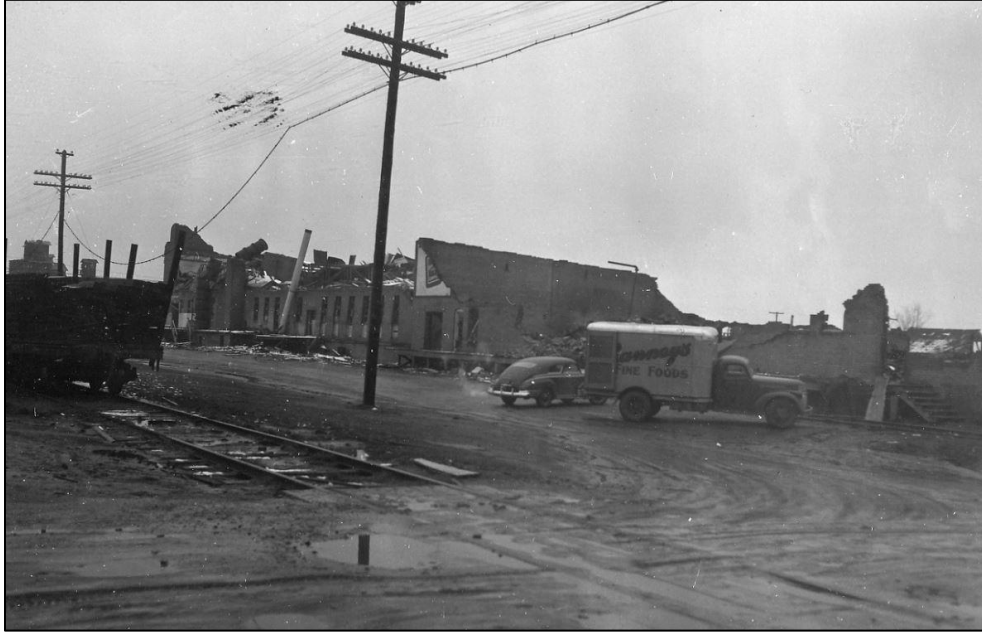
Figure 4: Tornado Damage in Woodward, OK 1947 (NWS n.d.)
