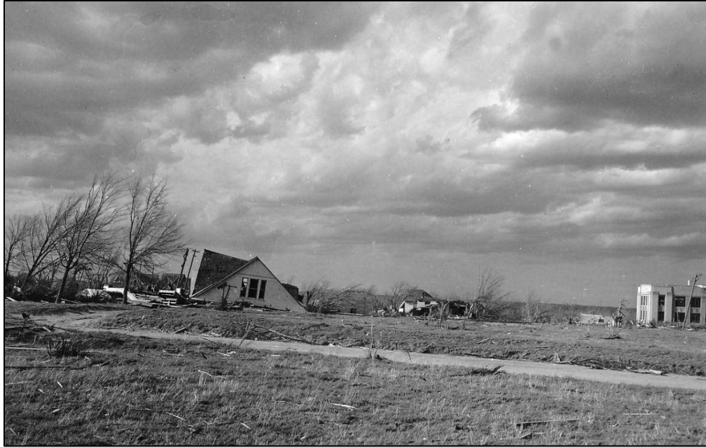
Figure 2: Tornado Damage in Woodward, OK 1947 (NWS n.d.)
