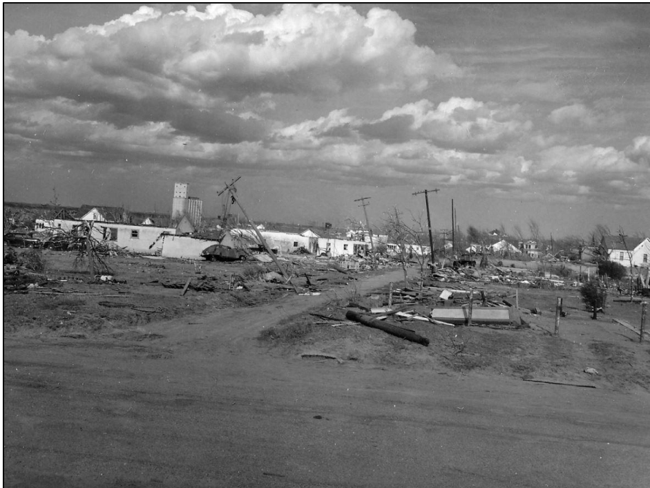
Figure 1: Tornado Damage in Woodward, OK 1947 (NWS n.d.)
