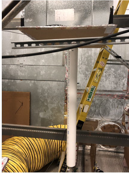
Figure A.19: Leak testing setup (unit side)
