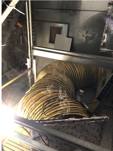
Figure A.21: Leak testing of flexible duct
