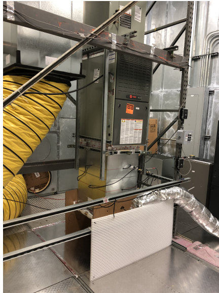
Figure A.8: Test setup with front air straightener
