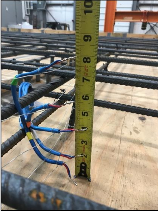
Figure 10. Installation of thermocouples on the bridge deck.
