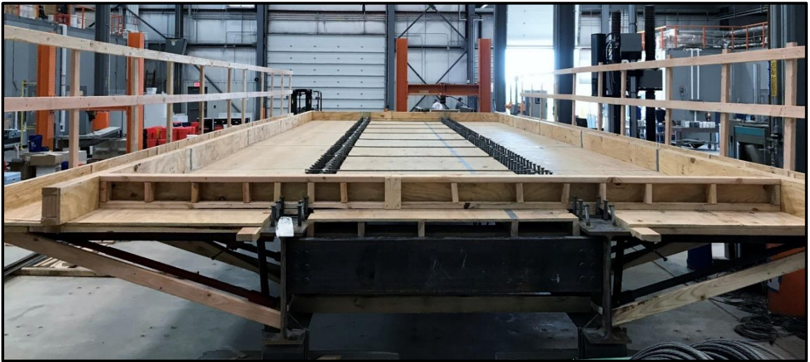
Figure 36. Laboratory Prototype Bridge built with formwork and bracing. View Looking East
