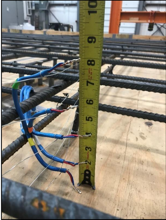
Figure 74. Installation of Thermocouples in concrete deck at mid-span
