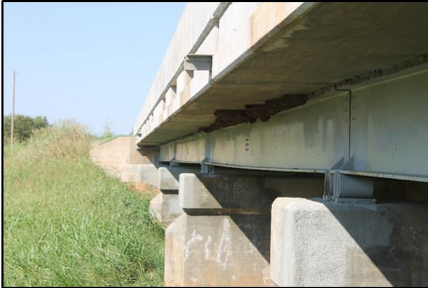
Figure 27. SH 14 Over Eagle Chief Creek, Bridge “A” in Woods Co.
