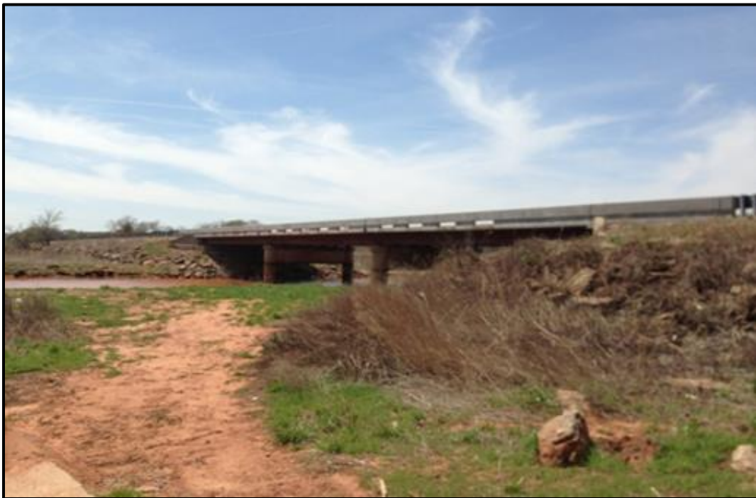
Figure 31. SH 86 over Stillwater Creek
