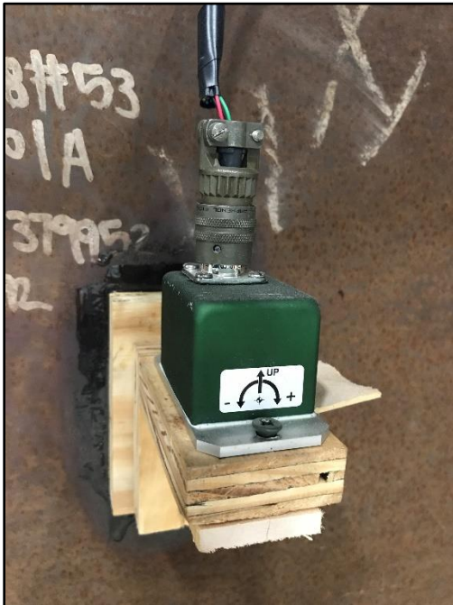
Figure 14. Installation of Jewell inclinometer on the steel girders
