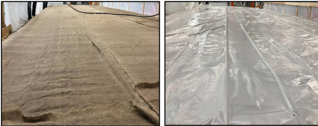
Figure 53. Wet burlap and 2 mil plastic was applied for 14 days
