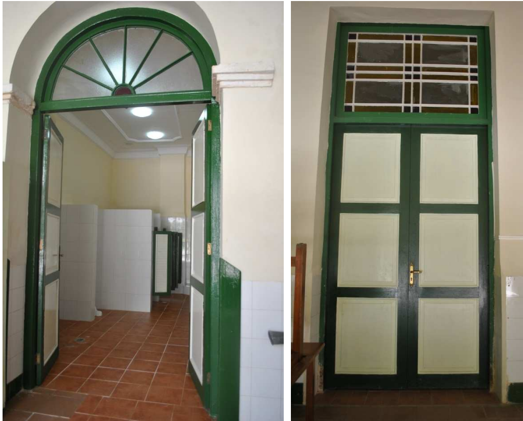
Figure 15: Restored doors, 2011 (Photo Credit: Author)
