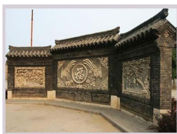
Figure 12: The Screen Wall
