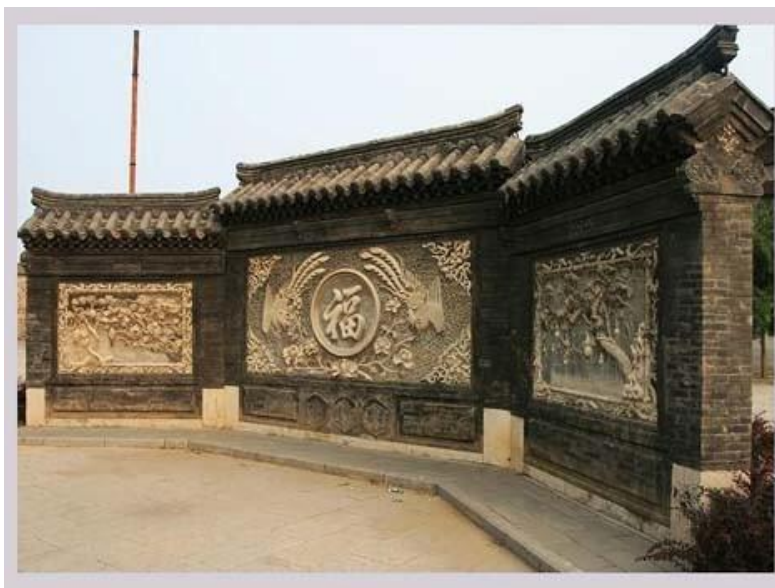
Figure 19: The Screen Wall
