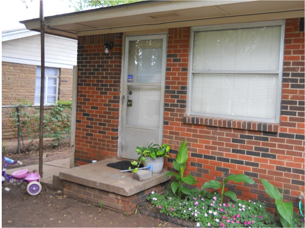
Figure 30: Photograph of outdoor living area (back porch)
