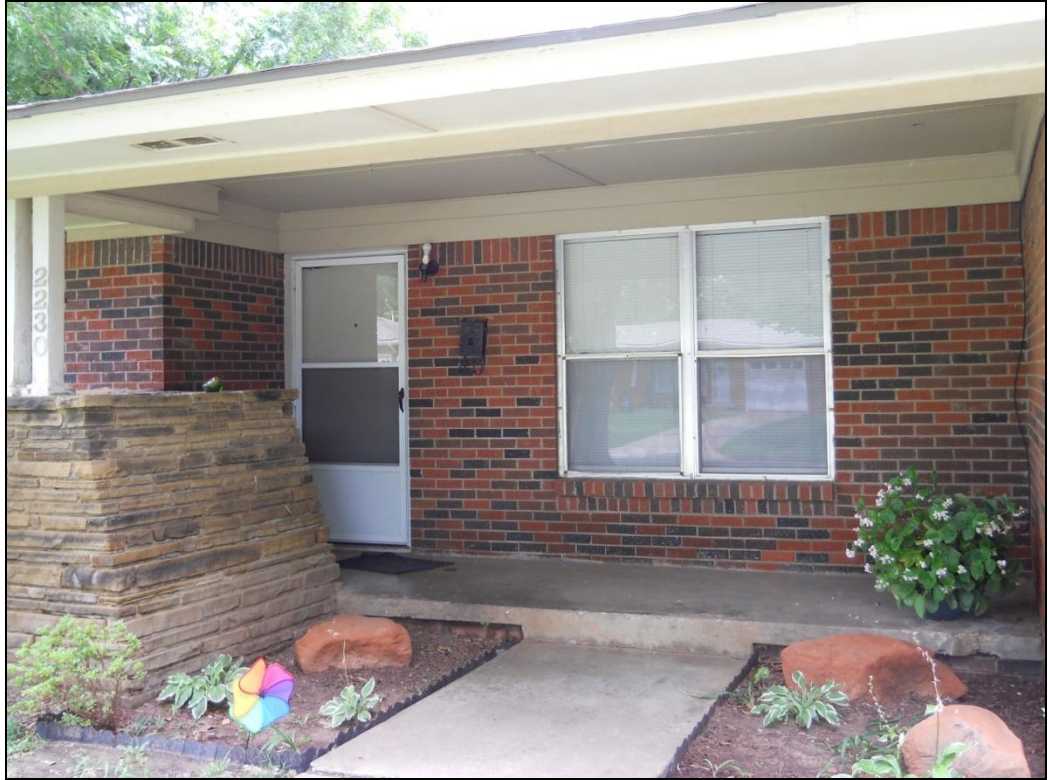
Figure 24: Photograph of front entry
