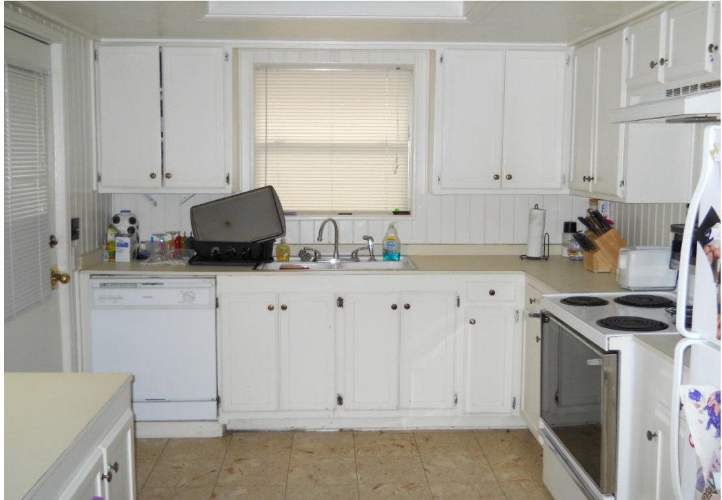
Figure 9: Photograph of kitchen illustrating assessment instrument violations due to an inaccessible sink, appliances upper cabinets, the lack of an interior laundry facility and a slippery floor
