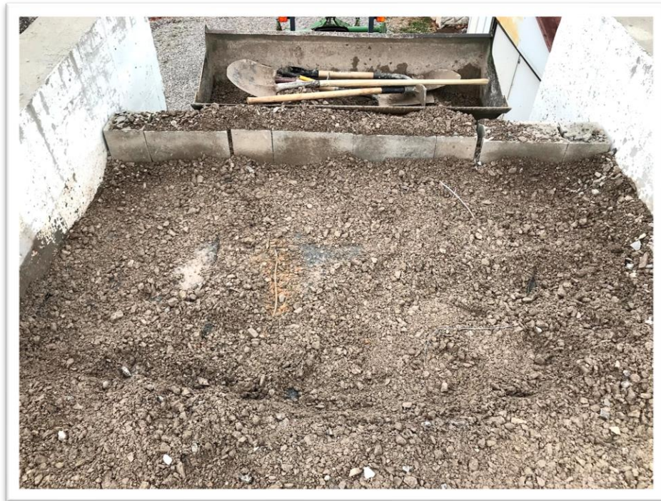
Figure 26 – Top GRS layer being excavated
