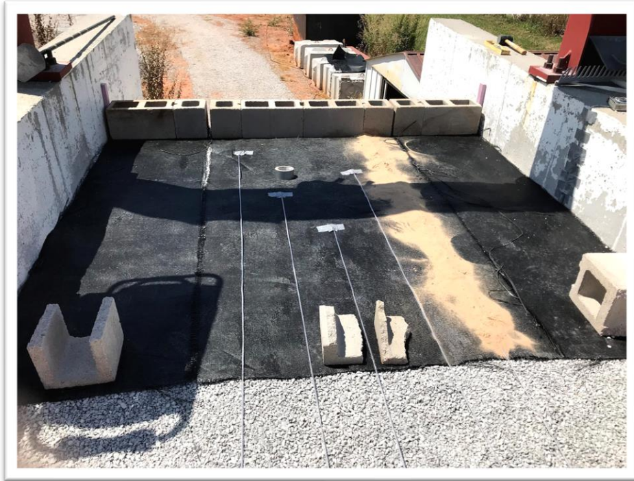
Figure 5 – Wire potentiometers being installed on one of the GRS abutment models
