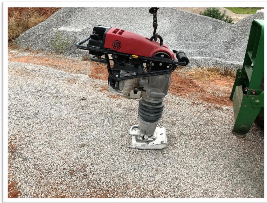
Figure 3 – Jumping jack used for the compaction of GRS fill
