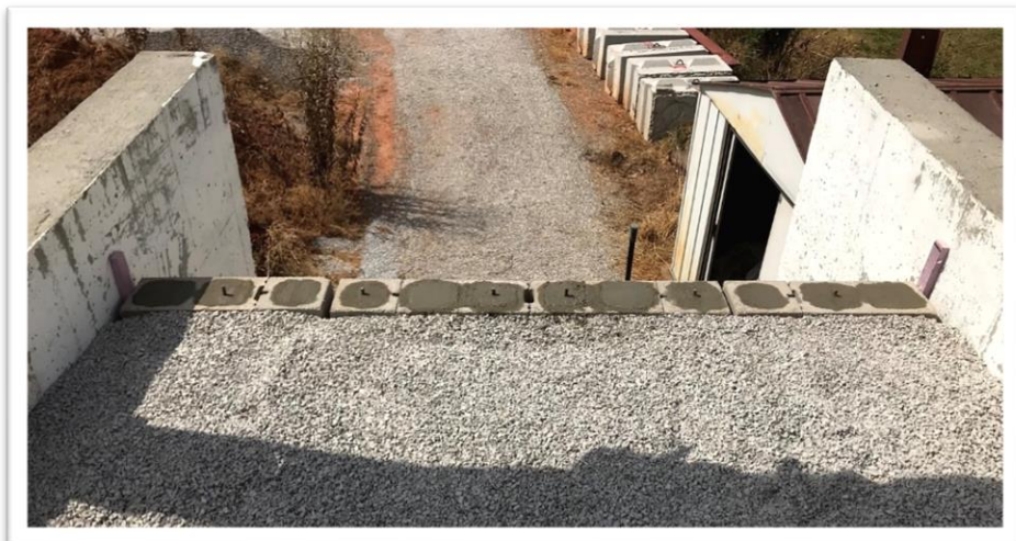
Figure 23 – Top three courses of CMU infilled with rebar and concrete
