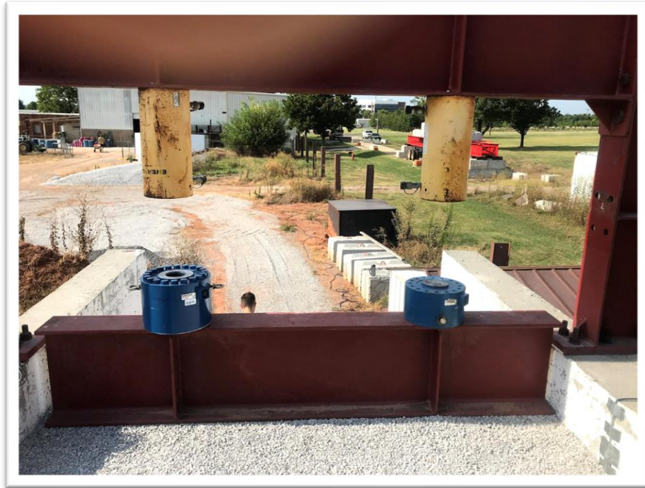
Figure 7 – Load cells (blue) on the loading beam
