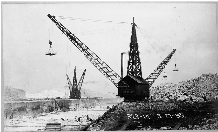
Figure 10: Lift Cranes along the Canal Ditch, 1895. Image Courtesy of the Encyclopedia of Chicago.
