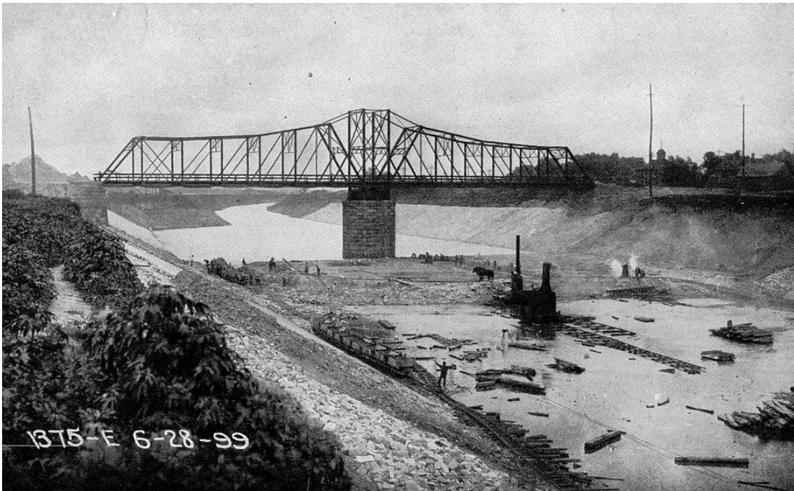
Figure 9: New Bridge Crossing the Canal Ditch, Looking East, 1899. Image Courtesy of F.E. Compton and Co. (1914), Chicago Historical Society.
