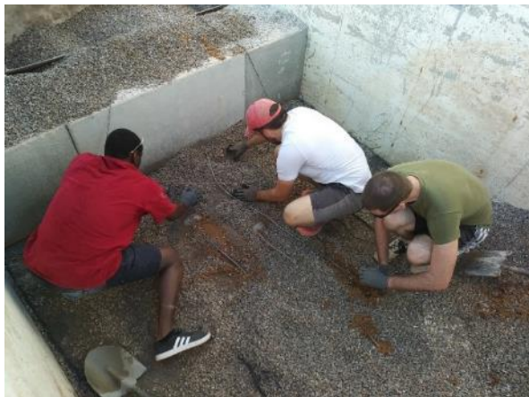
Figure 66. (Left) Instrumented reinforcement at the elevation of 27-inch above the foundation slab; (Right) EPCs located under the first-row of large concrete blocks in GRS Abutment Models #2 and #3
