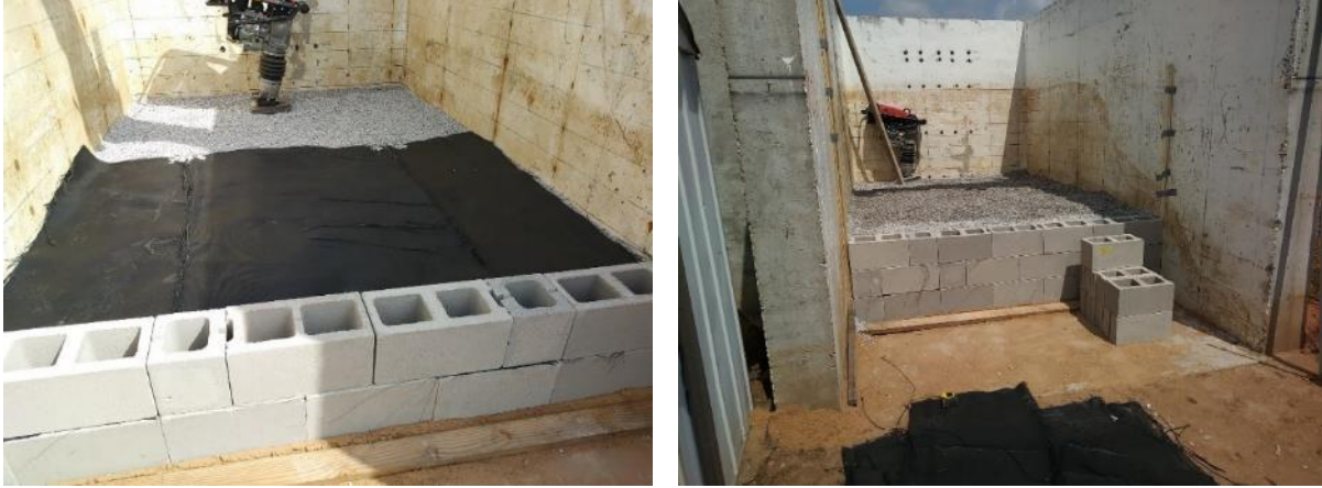
Figure 35. (Left) Placement of the second-row of CMU blocks; (Right) Third-row
