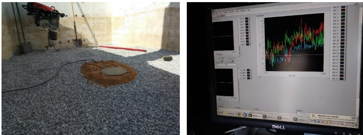
Figure 39. (Left) Installation of the fourth EPC; (Right) Readings from the WPs
