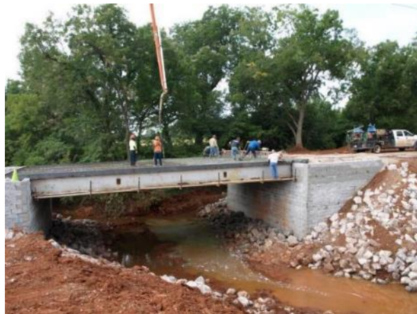
Figure 3. (Left) Condition of the old bridge; (Right) New GRS bridge abutment with CMU block facing in Lincoln County, OK, (Photograph courtesy of Mr. Tom Simpson)
