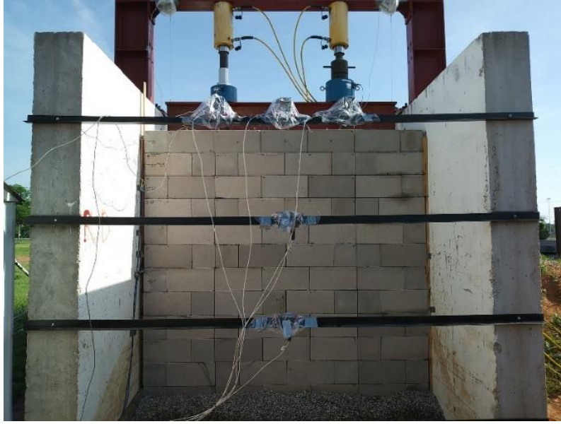
Figure 44. Installation of five WPs to measure facing deformation at different levels
