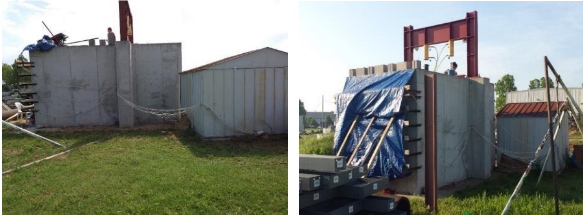
Figure 42. (Left) View from West side of the test station of WPs and the connecting cables to DAS housed in the shed; (Right) Back view
