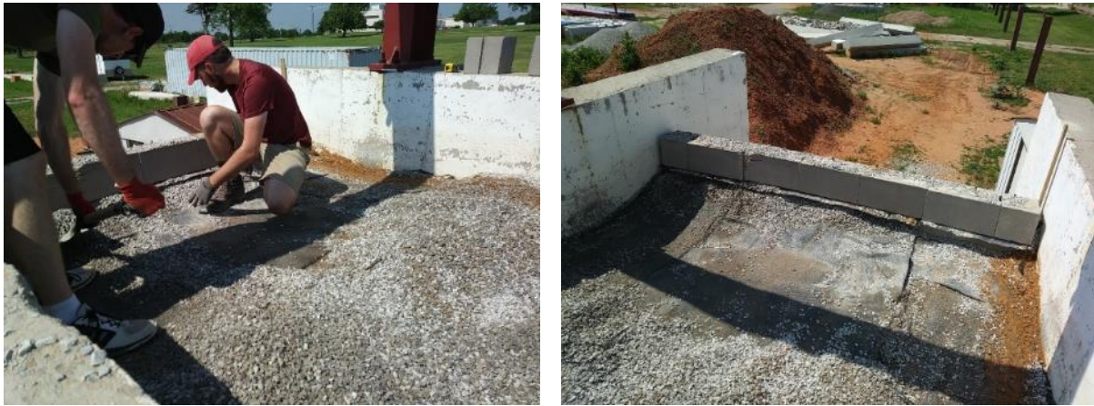
Figure 61. (Left) Layer by layer manual excavation of GRS Abutment Model #1 backfill; (Right) Observed geotextile deformation
