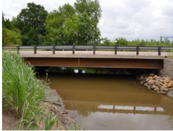
Figure 2. (Left) Condition of the old bridge; (Right) New GRS bridge abutment with CMU block facing in Kay County, OK, (Photographs Courtesy of Mr. Tom Simpson)
