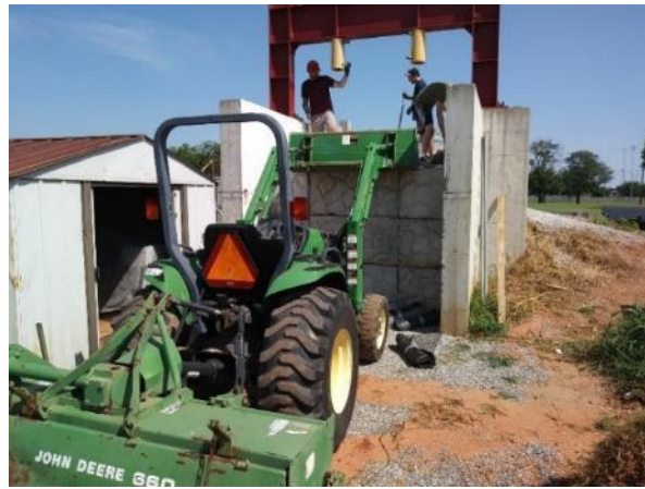
Figure 65. (Left) Removal of the large concrete blocks using a large forklift; (Right) Excavation and removal of bridge abutment gravel using shovels and a tractor
