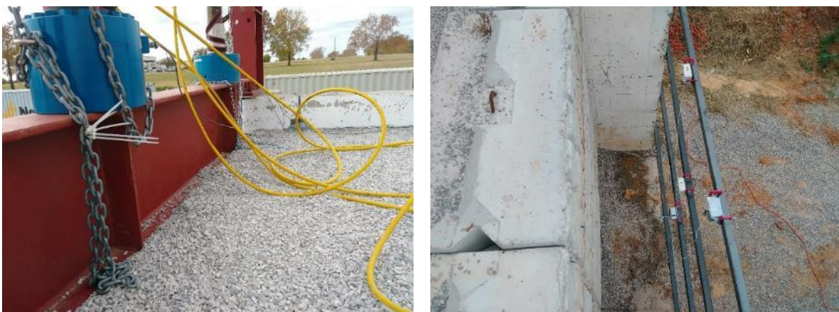
Figure 87. (Left) Back view of the loading beam after GRS Abutment Model #3 surcharge load testing; (Right) The top view of facing after the end of surcharge load testing
