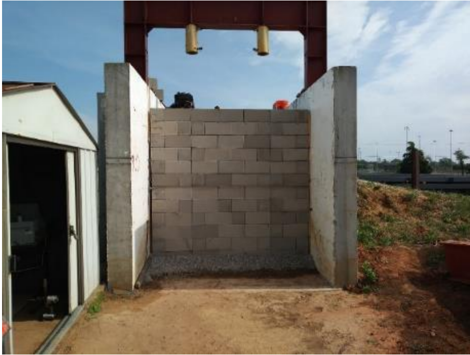
Figure 41. GRS Abutment Model #1 at the end of construction
