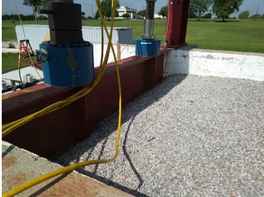
Figure 84. Settlement of the loading beam on the top of the GRS fill at the end of surcharge load testing of GRS Abutment Model #1
