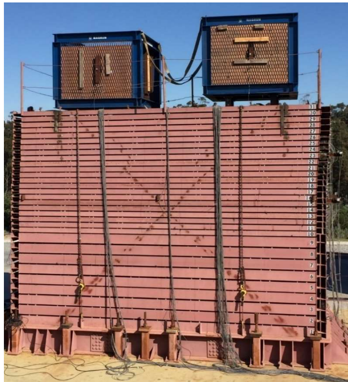
Figure 3.9. Grouped piles with sand-filled skid load on Day 4 and 5 of test
