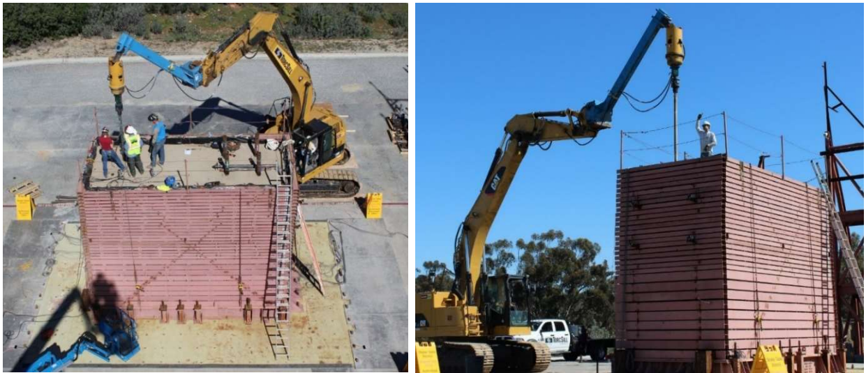
Figure 3.5. Pile installation image at UCSD
