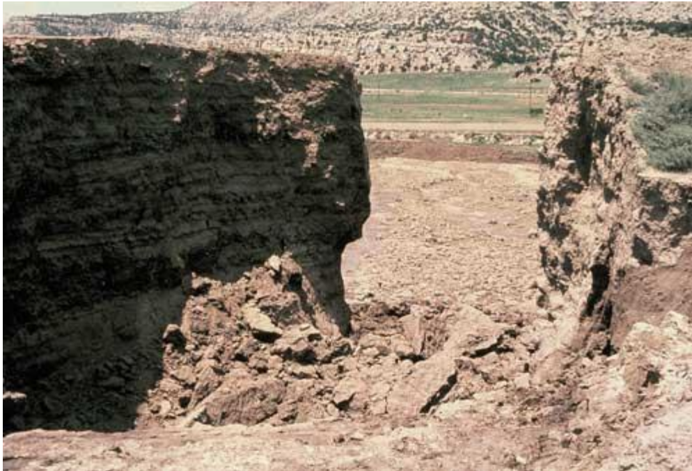
Figure 14: The breach at the Church Rock Uranium Dam. n.d. Photograph courtesy of the U.S. Environmental Protection Agency.
