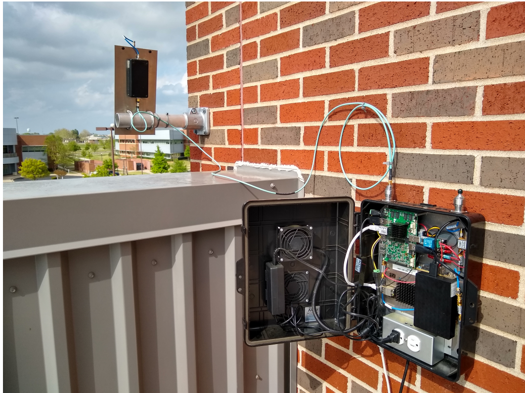
Figure 3.17: An installed system on the roof of the Radar Innovations Lab at the University of Oklahoma.
