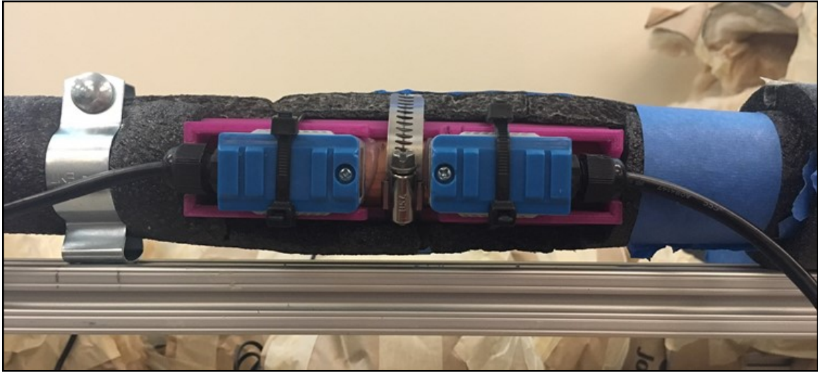
Figure B.3: Mounted transducers, using custom 3D-printed alignment tool (front view).
