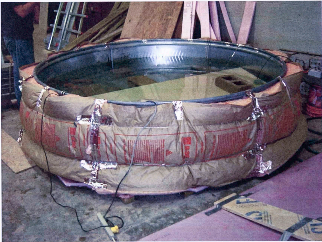
Figure 15 - Stock Tanks for Curing
