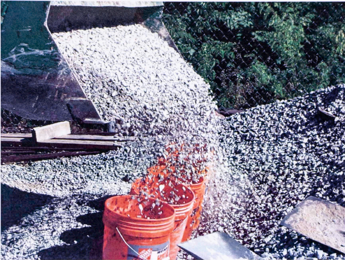
Figure 17 - Bucketing Aggregate Using a Front End Loader
