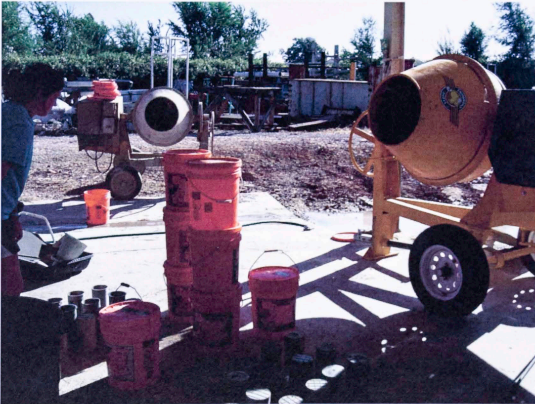
Figure 20 - Cylinder Molds and Material Ready for Batching
