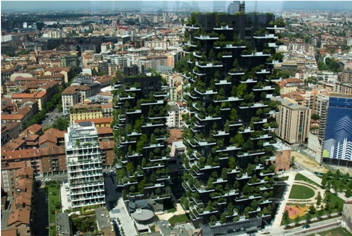
Figure 3.1 Bosco Verticale - Milan, Italy - Example of Building Integrated Vegetation
