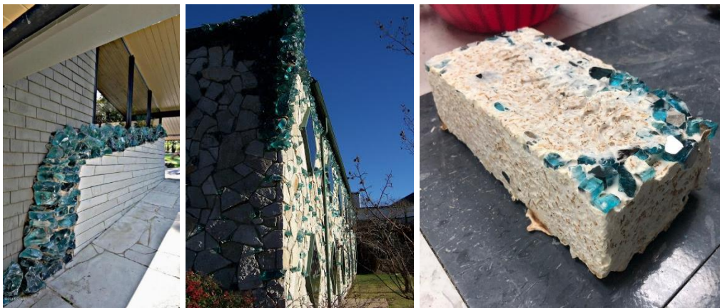
Figure 26: Illustration showing similar uses of blue “culled” recycled glass: Christ Redeemer Church designed by Bruce Goff in Bartlesville, Oklahoma, and the glass brick grown in lab
