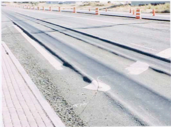
Figure 1.1: A Photographic View of Field Rutting
