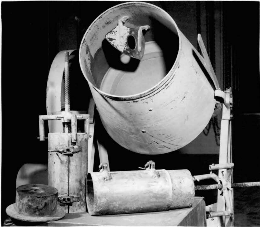
Concrete Mixer and Casting Molds
