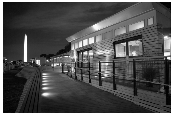
Fig. 1: The UWM Solar Decathlon project, on site in Washington, D.C. October 2009. Courtesy of Joseph Rice, UWM Solar Decathlon.
