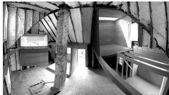
Fig 3 Interior view during construction.
