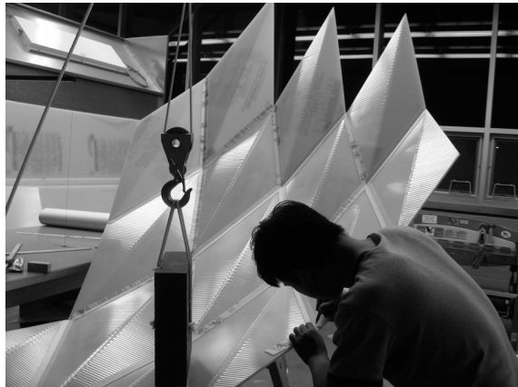
Fig. 7. Buffalo Bayou Origami Shell: Development of Folded Plate Panels. Photo by S. R. Perez.
