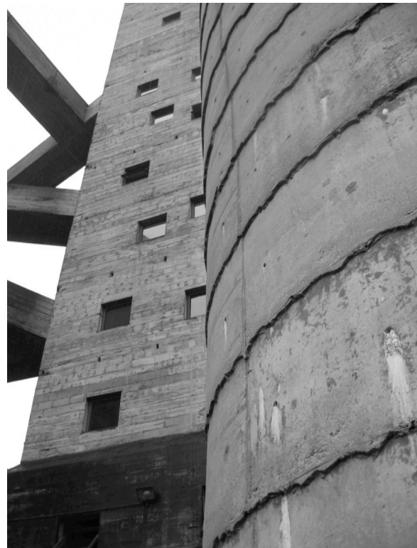
Fig. 5 SESC- Pompéia. View of water tower , locker room tower and elevated walkways to gymnasium tower. Photo by A. Ryba, 2005.
