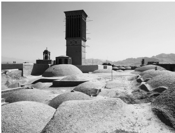
Fig. 11. Rooftop, Ganj Ali Khan Complex (photographed by Khosrow Bozorgi).
