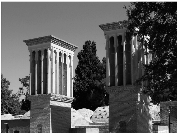
Fig. 12. Wind catchers, Shrine of Shah-Nimatota Vali, Mahan, Kerman (photographed by Khosrow Bozorgi).
