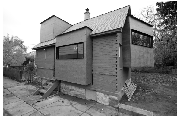
Fig 5 Back facade of 139 Howell St, Buffalo, New York.
