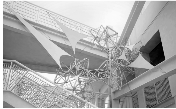
Fig. 12. Space frame with suspended cloth elements. (Image by Benson, D'Angelo, Darling, Emar, Morrow, Piccone, Siegel, Tait.)
