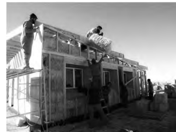
Fig. 12. Insulating Rabbit Ear House with hay, Navajo Nation, Utah, 2013.
