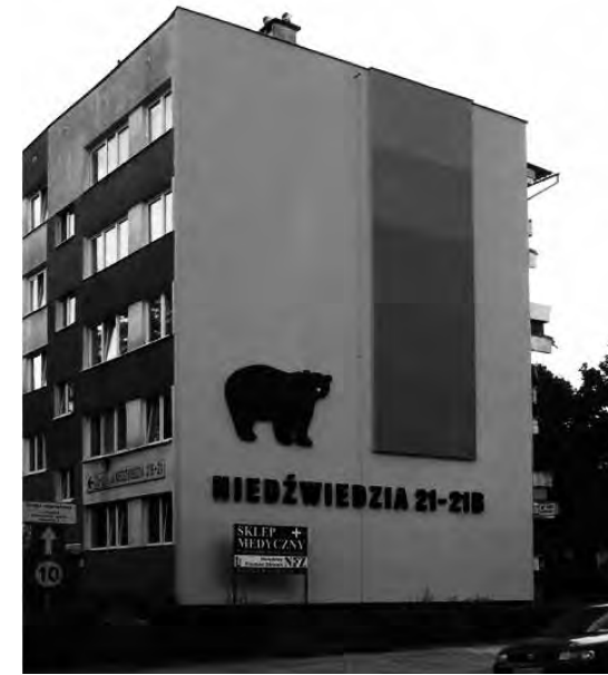
Fig. 4. Environmental signage applied to an end elevation of a five-story row house building.
