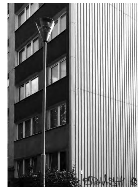
Fig. 5. The results of thermal insulation upgrades on adjacent elevations.
