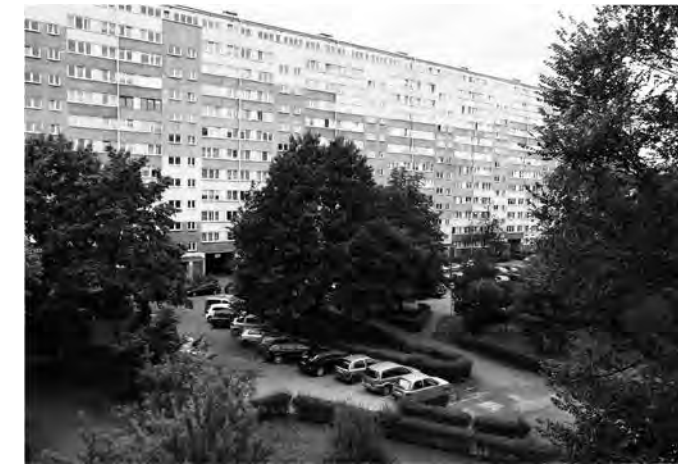
Fig. 1. Typical 1970s high-rise building. Socialist large block estate in Wroclaw, Poland.
