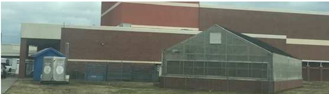
Figure 20. An empty and unused greenhouse at school site K.
