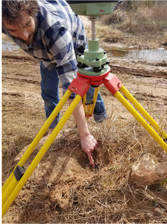
Figure IV.23: GPS base station.
