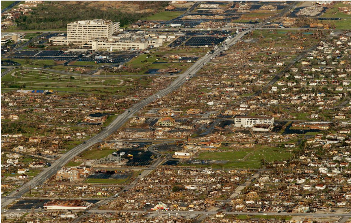
Figure 3. Damage to a Joplin Residential Area (Riedel 2011)
