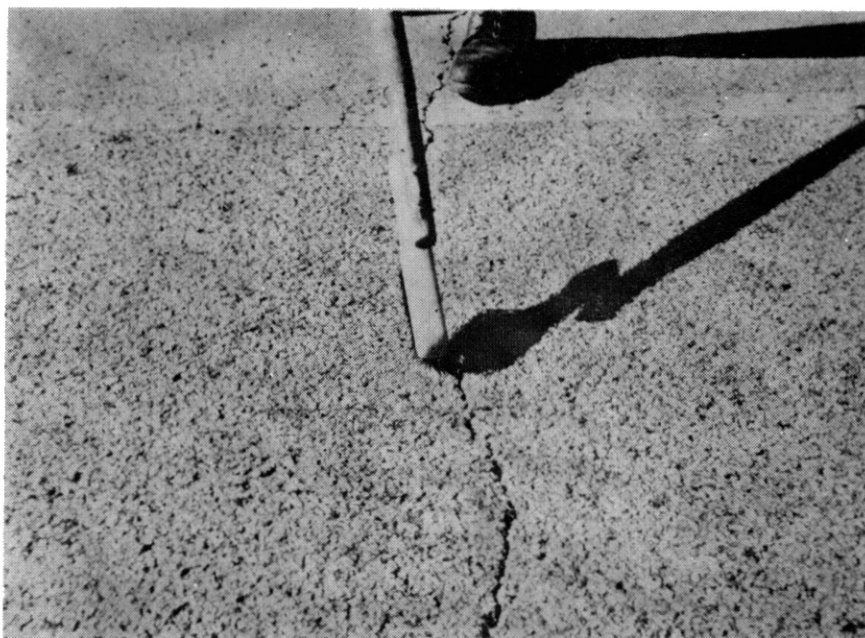
Figure 10. Brushing Transverse Crack Prior to Air-Blowing.
