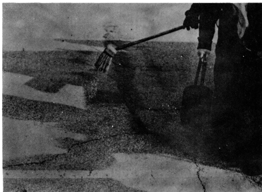
Figure 13. Application and Sanding of Emulsions.
