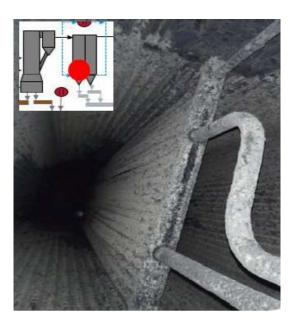
Figure 1.8. The thin layer of dust in the boiler after operating for 13000h with syngas [35]
