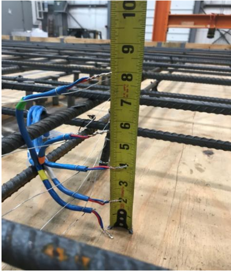
Figure 3.4 - Photograph of thermocouples used for data collection: Thermocouples were placed at the top and bottom surface of the deck and at 2in., 4in., and 6in. depths.
