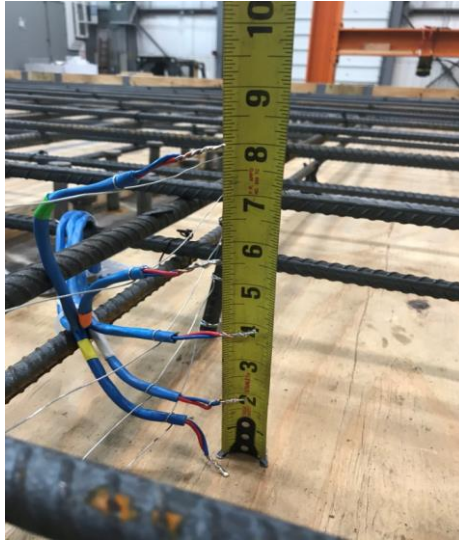
Figure 4.4 - Photograph of thermocouples used for data collection: Thermocouples were placed at the top and bottom surfaces of the deck and at depths of 2 in., 4 in., and 6 in.
