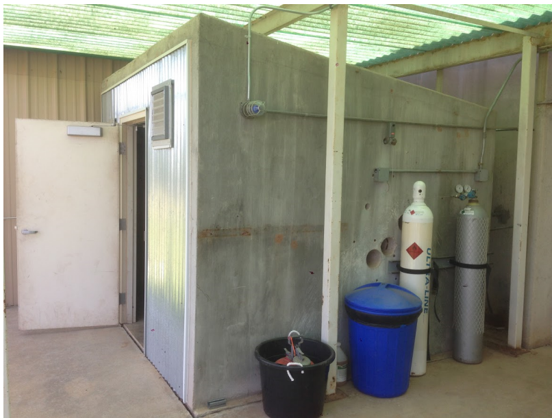
Figure 5.5: Exterior of the Hazardous Reactions Lab blast cell
