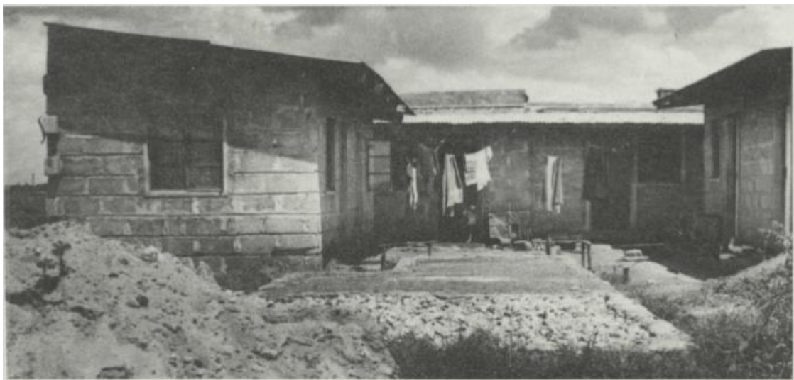
Figure 17- Average completed dwelling, with a planned extension and constructed ground-floor slabs. (Source: Praful Soni, 1981)
