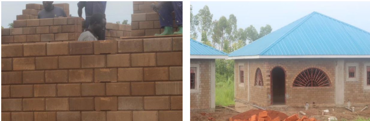
Figure 5- Examples of buildings made from compressed earth block [CEB] from Atiak, Uganda. (Source: Author)
