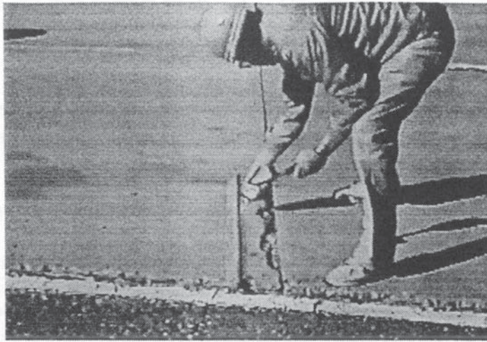
Figure 16. Marking of repair area.
