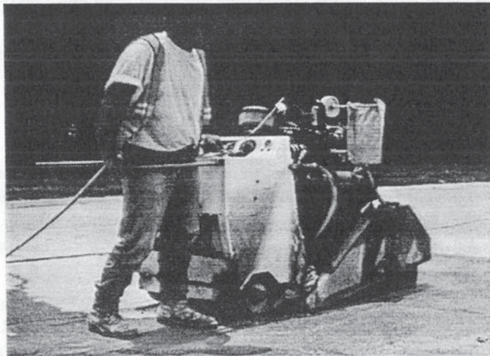
Figure 6. Full depth sawing operation.
