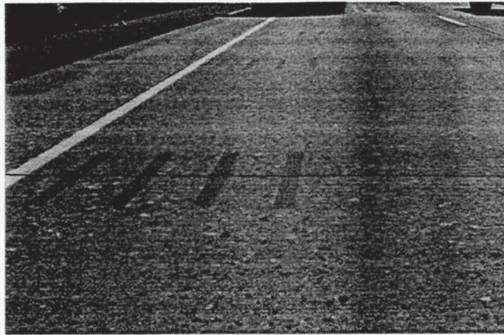
Figure 40. A completed load restoration project.
