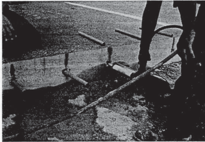
Figure 11. Epoxy resin injection into dowel holes.
