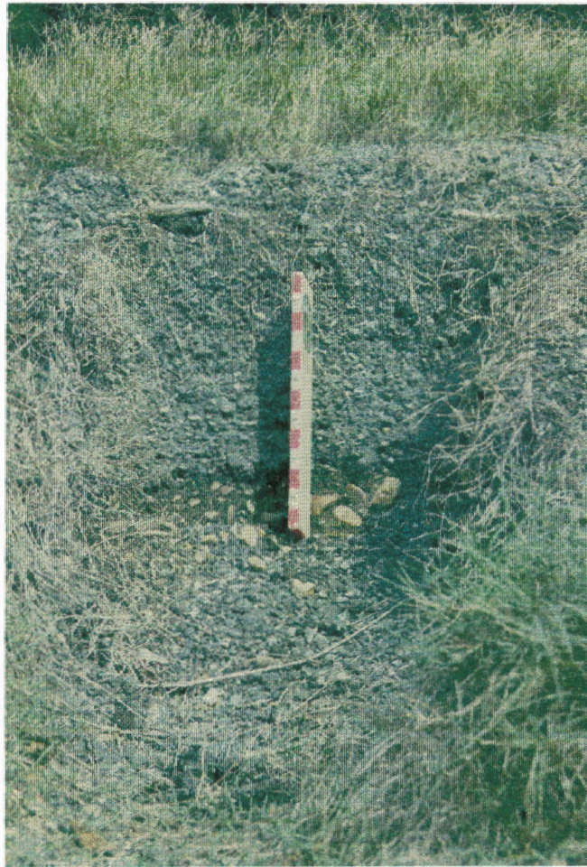
Figure 3.7 Millings Used for Erosion Control on SH 3 near Farris
