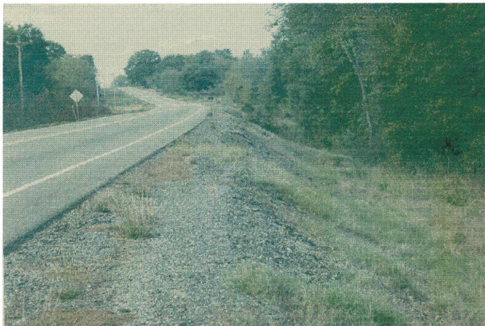
Figure 3.4 Millings Used for Shoulders on SH 3 near Farris
