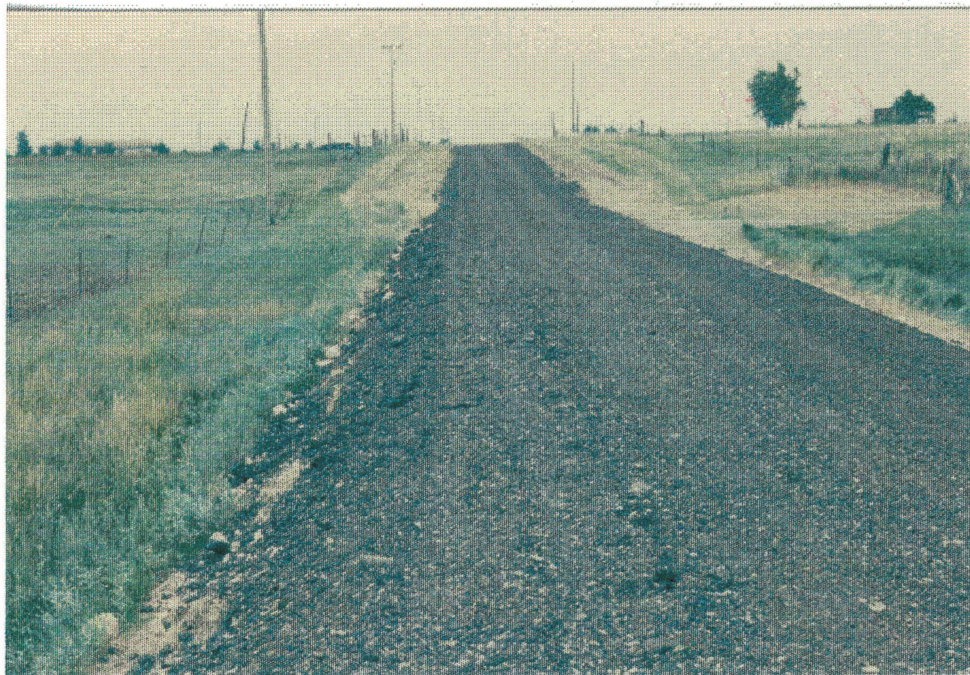
Figure 3.14 Millings Used as Base
