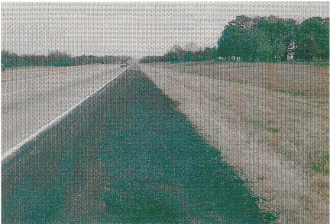
Figure 3.2 Untreated Millings for Shoulders on I-40 in Sequoyah County
