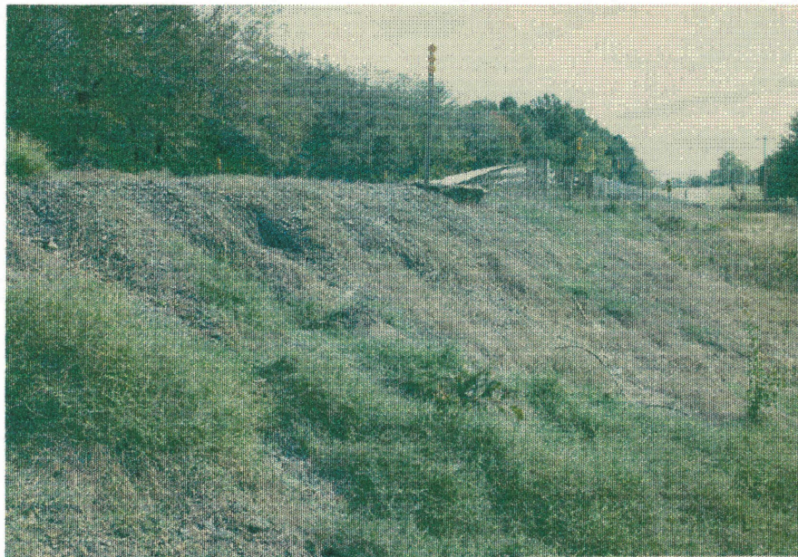
Figure 3.6 Millings Used for Erosion Control on SH 3 near Farris
