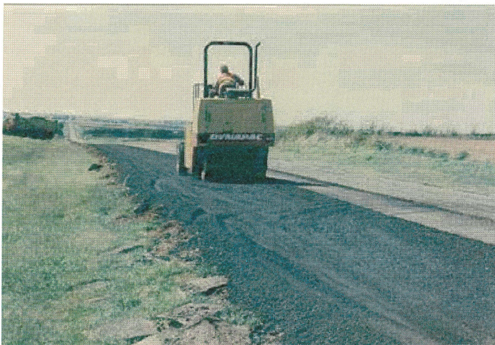
Figure 3.16 Pneumatic Compaction of Processed Millings on US 60
