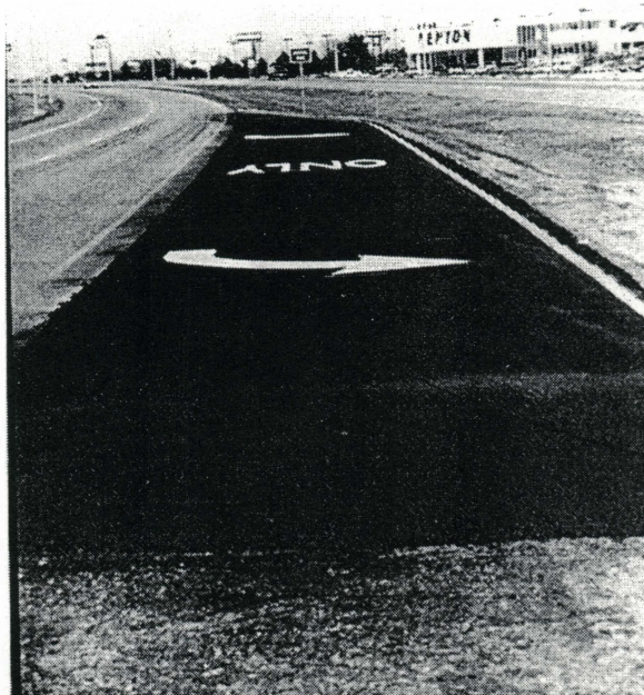
Figure 3.3 Millings Used as Base Material on McAlester, US 69 By Pass
