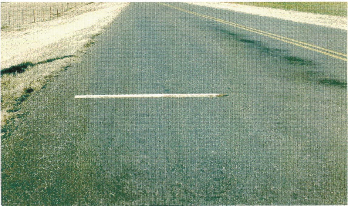
Figure 3.12 75mm Thick Surface Course on SH 183 A near Bessie
