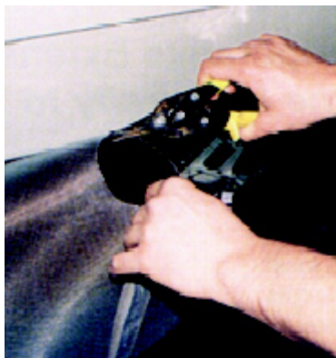
Figure 9B. Cut away excess screening to accommodate trap top assembly.
