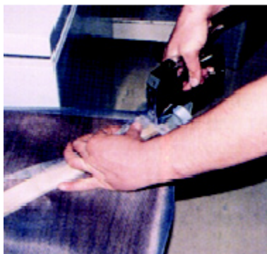
Figure 9D. Anchor trap top between screening and wood lath and staple in place.
