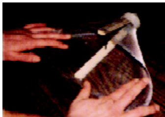
Figure 6G. Anchor dry wall screw into larger piece of wood lath. Do not go through the wood.
