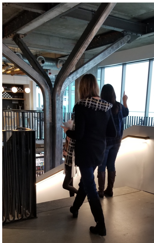
Image 13: Monumental Stair Structure at Little
