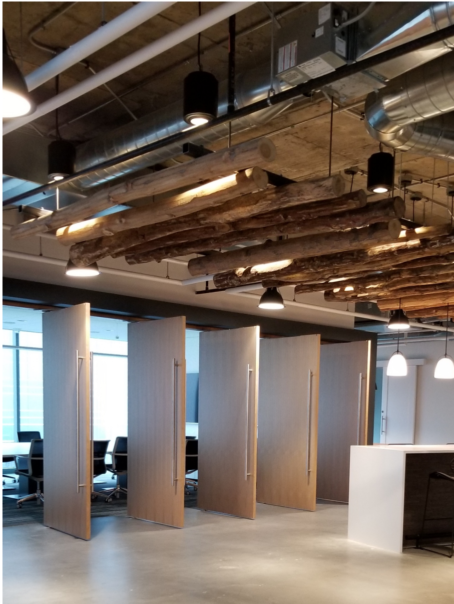
Image 15: Large Conference Room at Little
