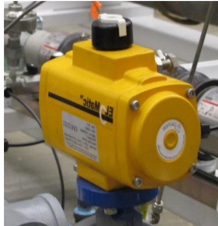
Figure C.5 Quick closing valves
