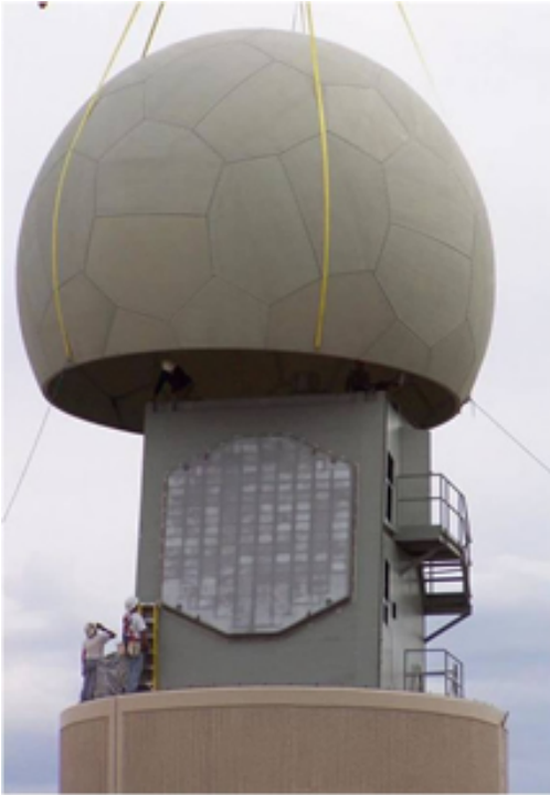
Figure 1.3: The NWRT PAR is a Navy SPY-1A converted for weather radar purposes.
