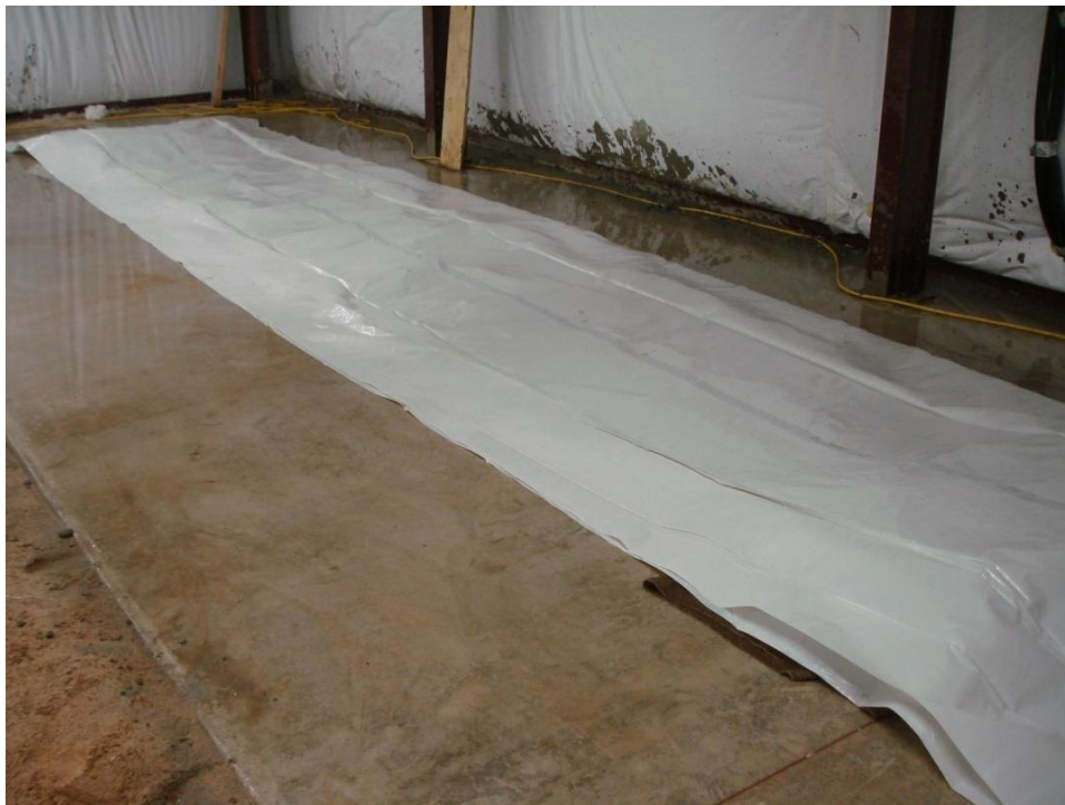
Figure 3.25 Moist cured slab
