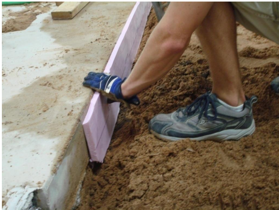
Figure D.2 Placing Foam around the slab specimens
