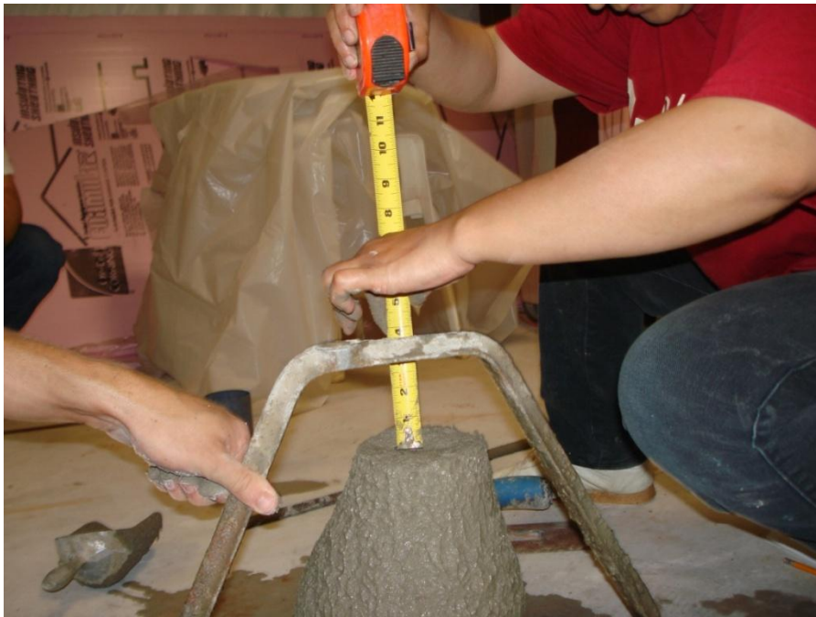
Figure D.15 Concrete slump measurement
