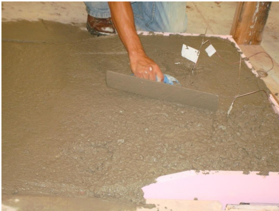
Figure 3.22 Finishing concrete surfaces at end of the slab
