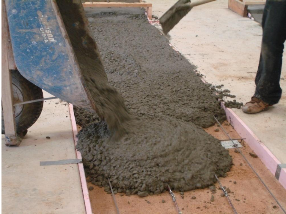
Figure 3.21 Casting concrete slab
