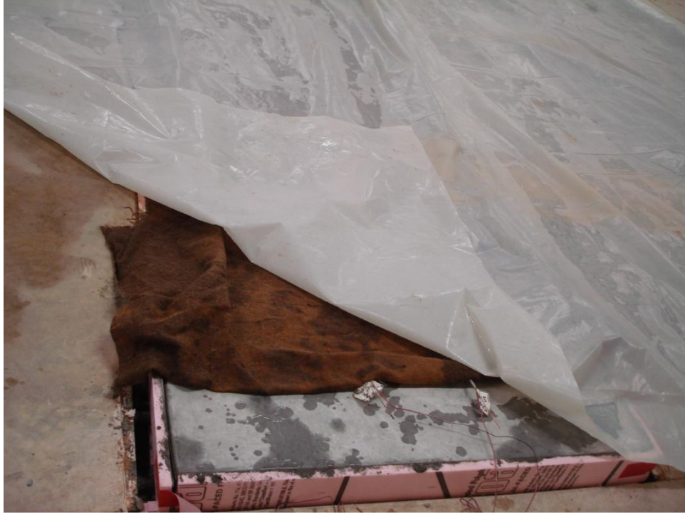
Figure 3.26 Wet burlap and plastic sheet used for curing concrete slab
