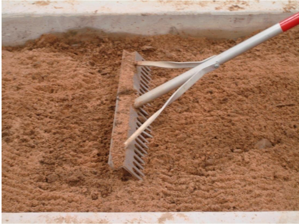
Figure 3.8 Making sand ready for slab on grade
