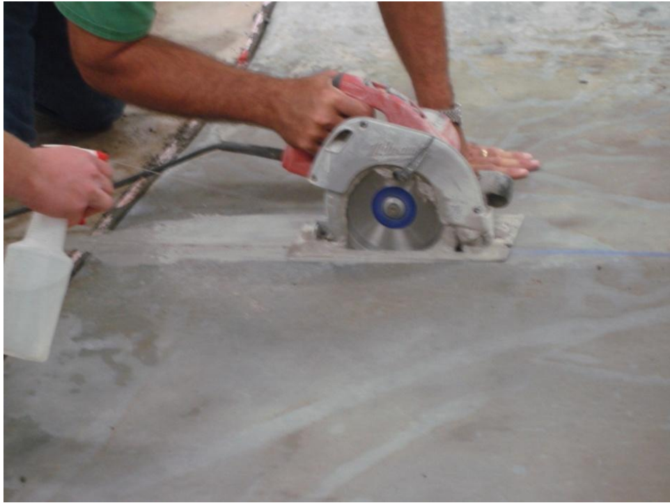
Figure 3.27 One inch sawcut joint
