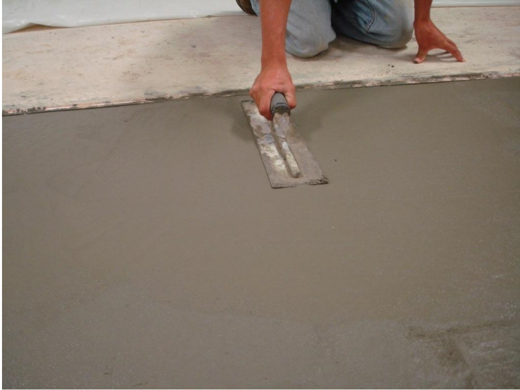
Figure 3.23 Finishing concrete surface
