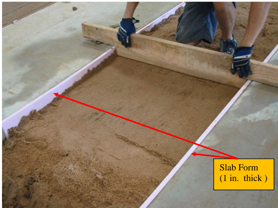
Figure 3.9 Four inches moist compacted sand
