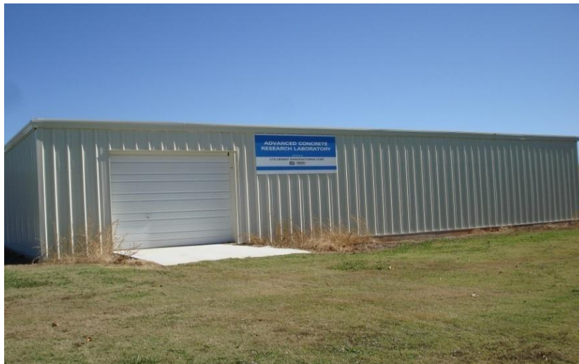
Figure 3.2 Exterior view of lab construction
