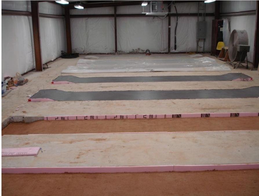
Figure 3.7 Interior view of Advanced Concrete Research Lab
