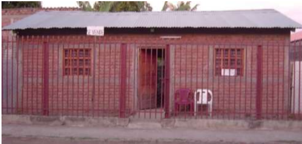
Figure 8.30. Confined masonry building in Rivas, Nicaragua
