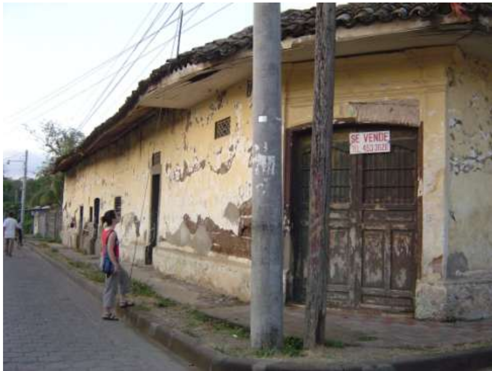
Figure 8.48. Taquezal building, Rivas, Nicaragua
