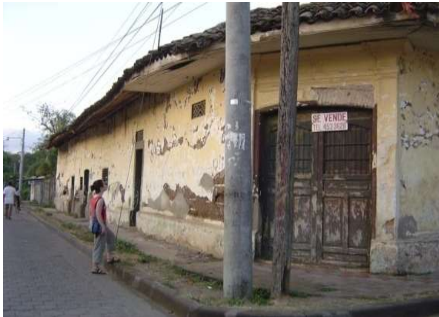
Figure 9.3. Taquezal building
