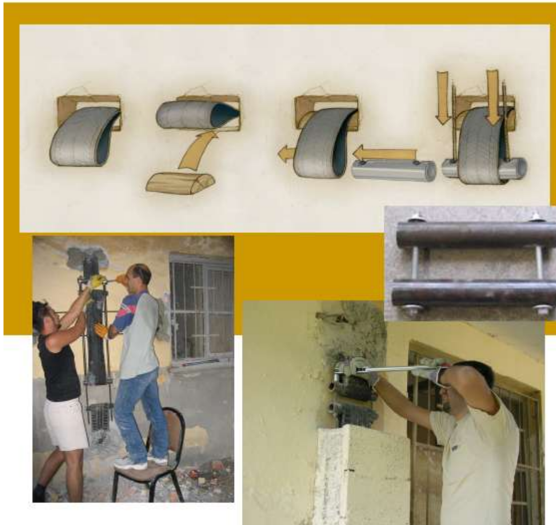
Figure 4.19. Building retro-fit using scrap tires (Turer, 2003)
