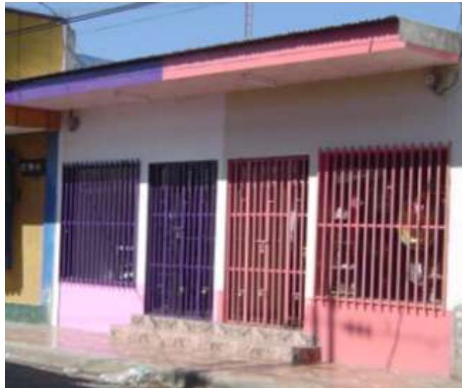
Figure 8.1. Typical concrete building chosen for analysis
