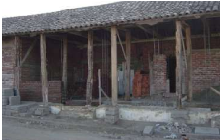
Figure 4.14. Retrofitting by removing taquezal walls and replacing with confined masonry
