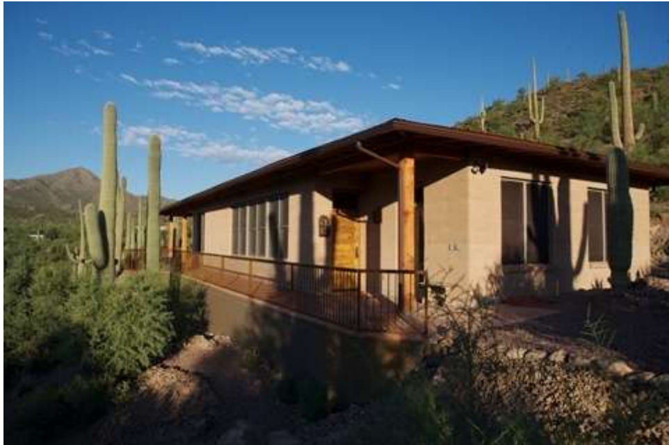
Figure 4.2. Rammed earth home in the Southwestern United States http://www.rammedearth.com/gallery.html
