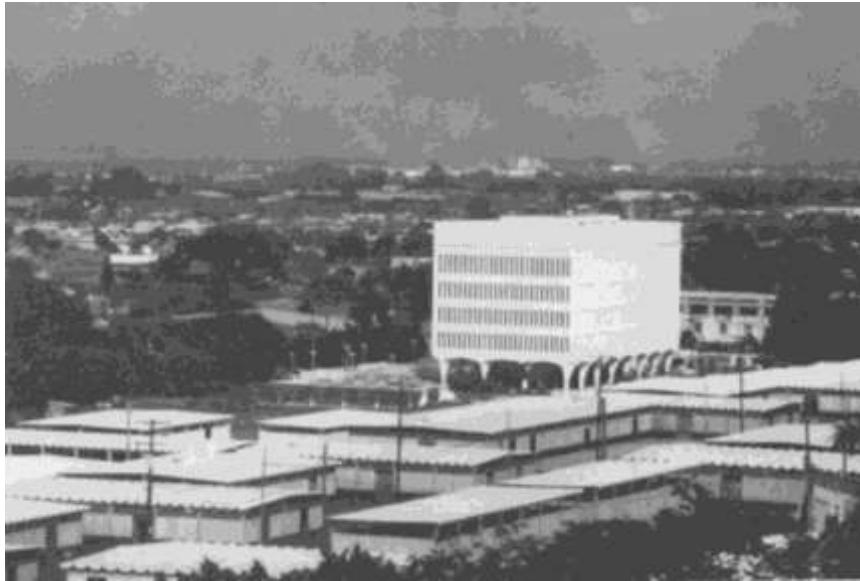
Figure 3.21. ENALUF (Light and Power) Building, notice the soft first story (Sozen and Matthiesen, 1975).
