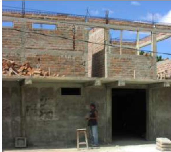
Figure 5.1. Confined masonry construction, San Juan del Sur, Nicaragua
