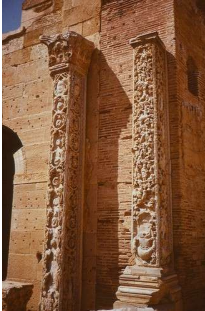
Figure 4.18. Photo of pilaster retrofit example
