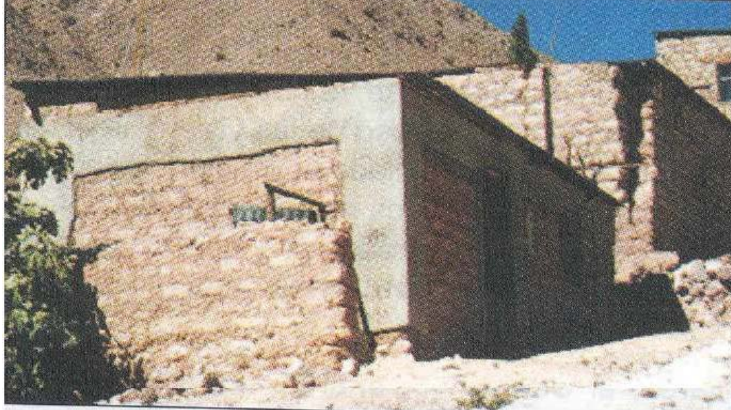
Figure 4.20. Rehabilitated adobe dwelling (San Bartolome, 2004)
