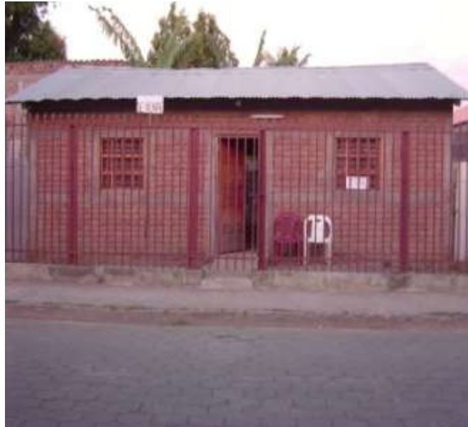
Figure 9.4. Confined masonry building
