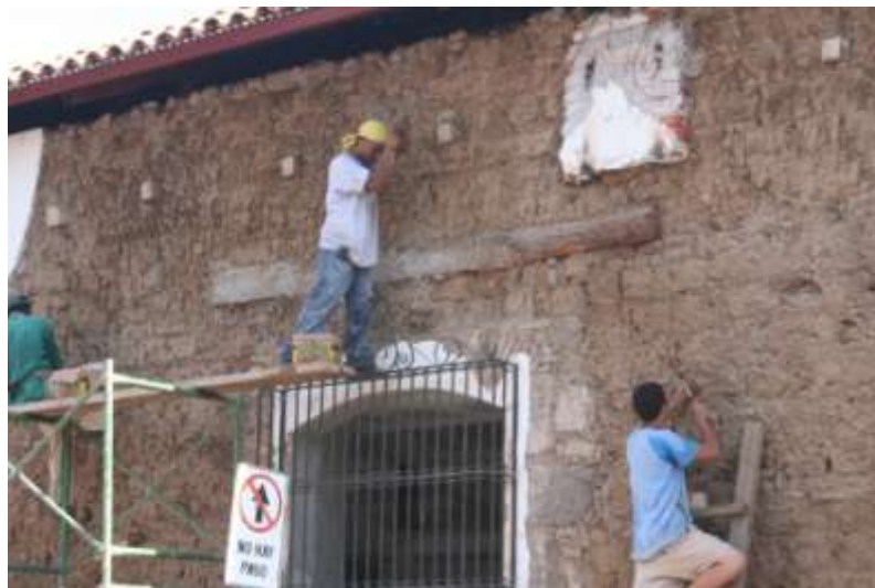
Figure 4.1. Adobe building in Leon, Nicaragua undergoing repairs
