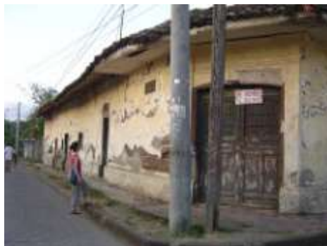
Figure 3.19. Taquezal construction, Rivas, Nicaragua
