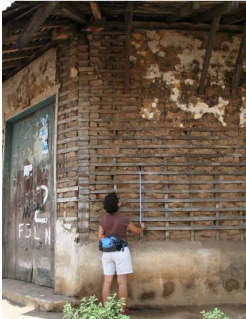
Figure 8.51. Typical taquezal framing used for model
