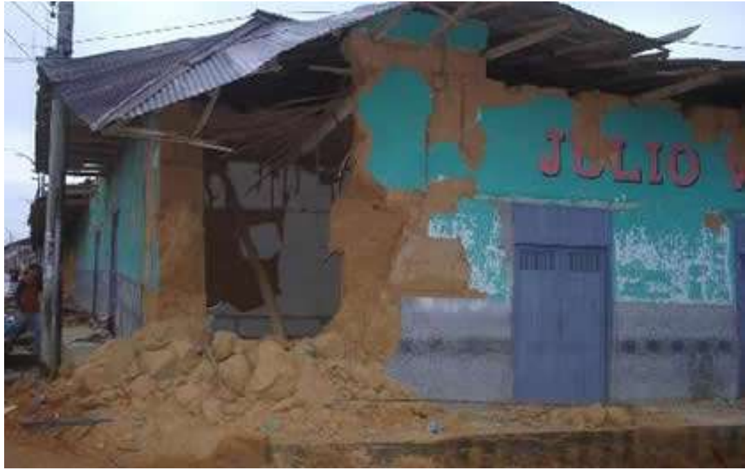
Figure 9.2. Rammed earth building (Diaz, 2007)
