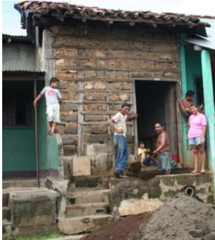
Figure 4.3. Taquezal house in Leon, Nicaragua undergoing repairs
