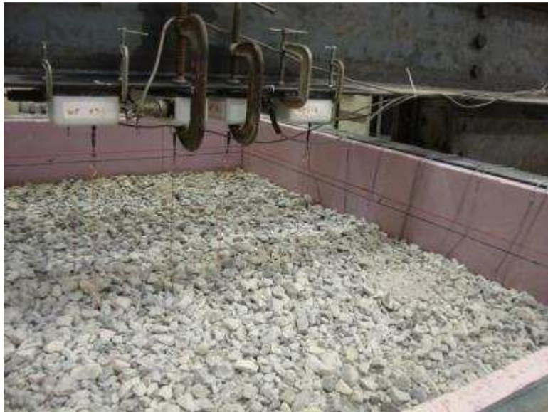
Figure 9.38. Compacted aggregate layer placed on the geogrid reinforcement
