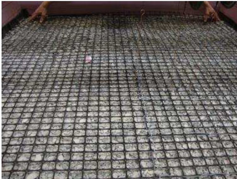
Figure 9.36. Placing geogrid reinforcement on the 25 mm-thick aggregate layer
