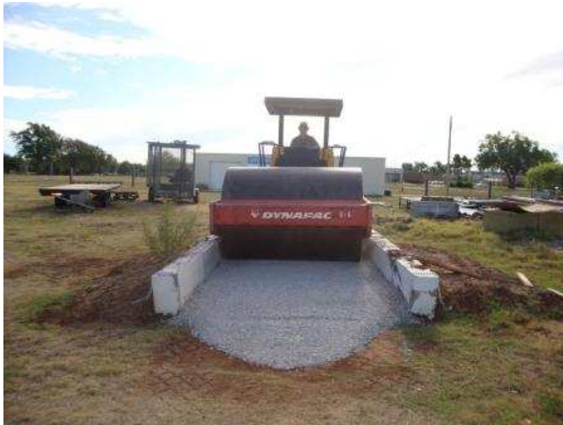
Figure 7.25. Compacting the first layer of aggregate with a vibratory roller compactor
