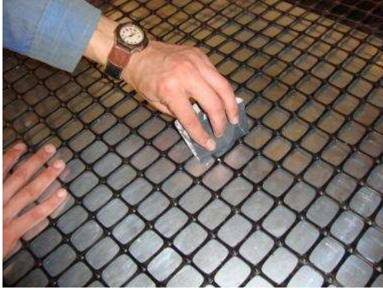
Figure 9.10. Abrasive paper was used to roughen the surface of the extruded geogrid
