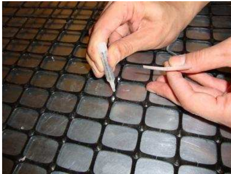
Figure 9.13. Application of adhesive material to the geogrid
