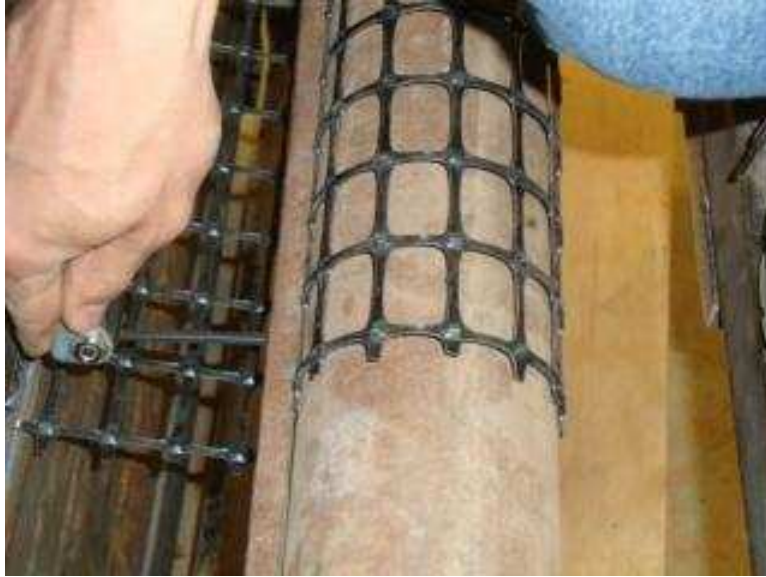
Figure 8.12. Geogrid was connected to the roller clamp
