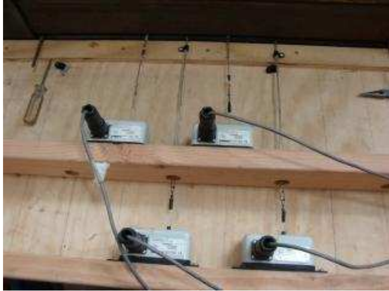
Figure 8.6. Tell-tale wires connected to wire potentiometers
