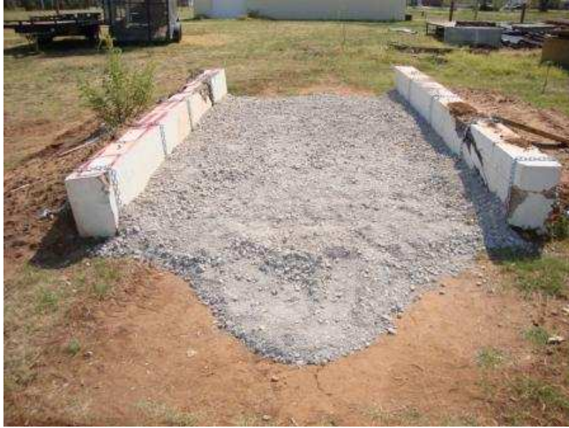
Figure 7.24. First layer of aggregate in the test bed before compaction
