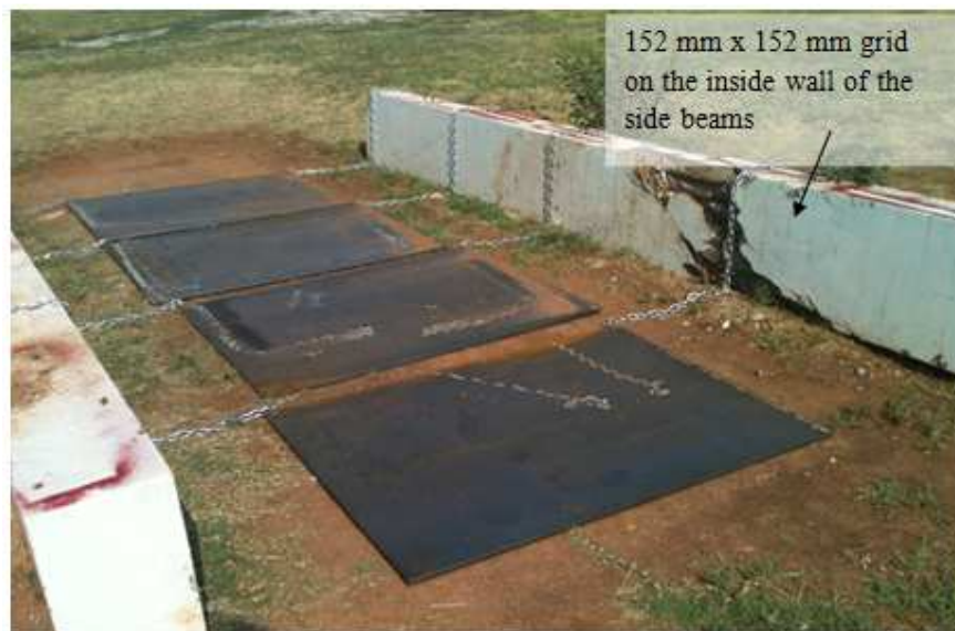
Figure 7.21. Four steel plates were placed in the test bed to facilitate the exhumation process of geogrids after they were covered by compacted aggregate
