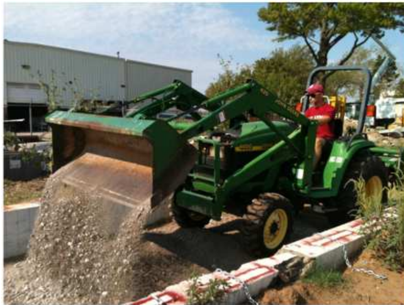
Figure 7.23. Spreading ODOT Type-A aggregate in the test bed
