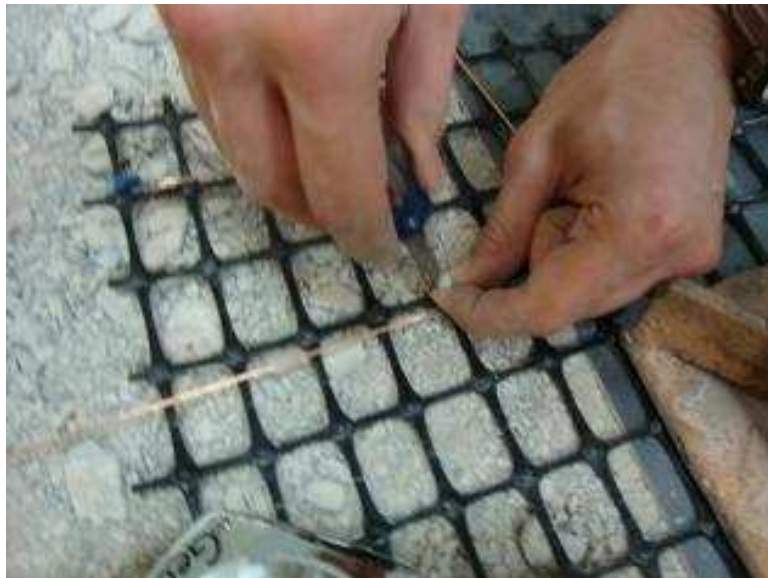
Figure 8.5. Connecting wires to geogrid specimen
