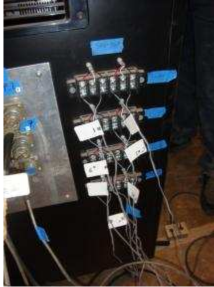
Figure 9.44. Eight strain gauges connected to the DAS
