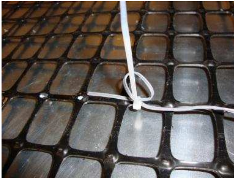
Figure 9.19. Wire tie was used to hold the strain gauge wire in position
