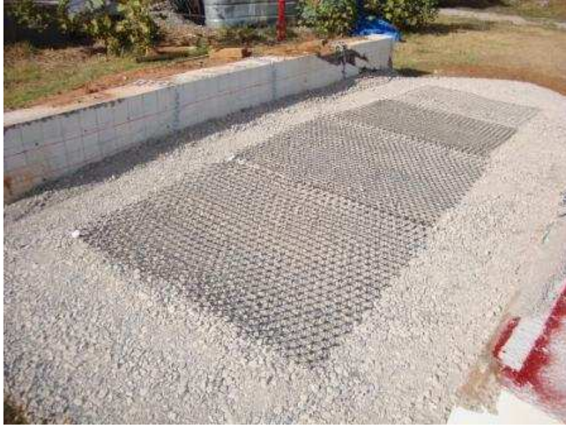
Figure 7.27. Four extruded geogrids placed on the first layer of compacted aggregate
