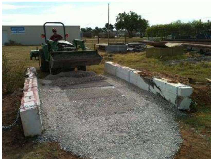
Figure 7.28. Spreading the second layer of aggregate in the test bed
