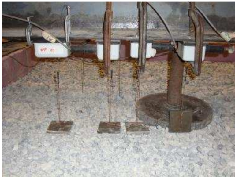
Figure 9.41. Setup of the telltale plates on the top of the aggregate layer
