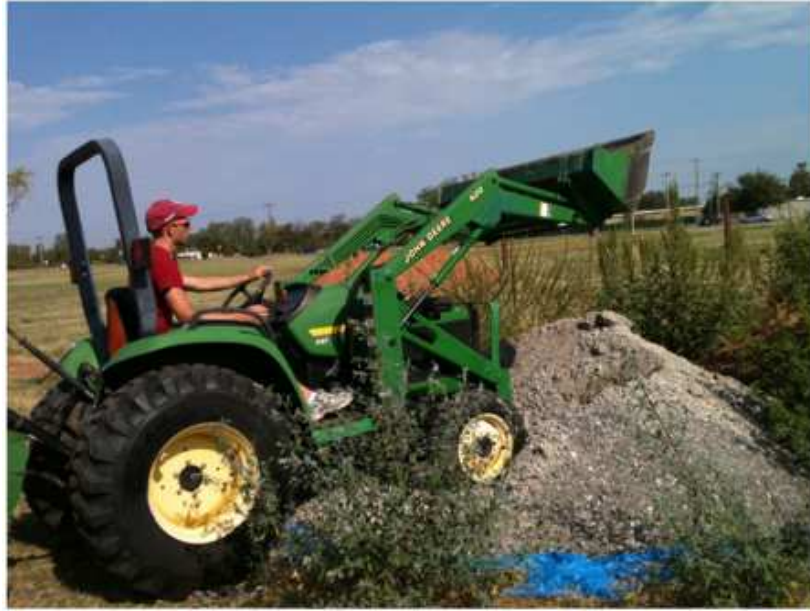
Figure 7.22. Aggregate was taken from a nearby stockpile using a front-loader tractor
