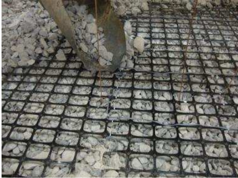
Figure 9.37. Careful placement of aggregate on the geogrid layer
