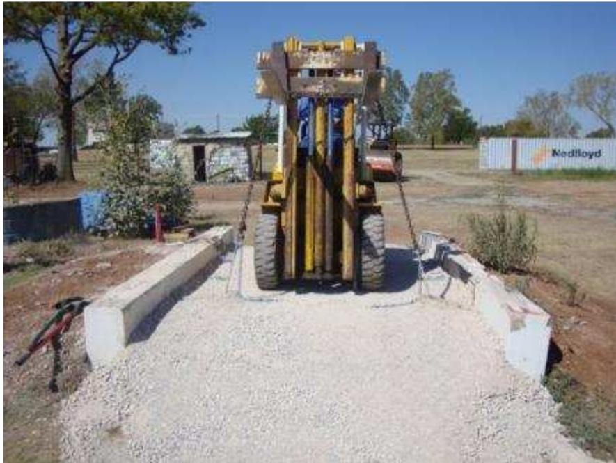
Figure 7.31. Forklift connected to the lifting chains
