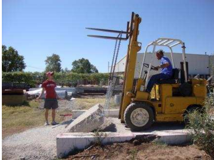
Figure 7.32. Tilting of steel plates from underneath the compacted aggregate
