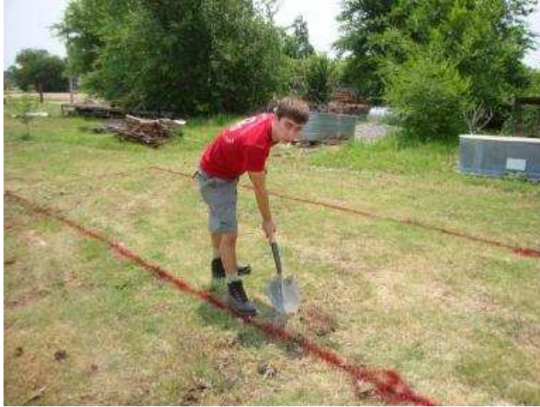
Figure 7.19. Clearing the test area from existing vegetation
