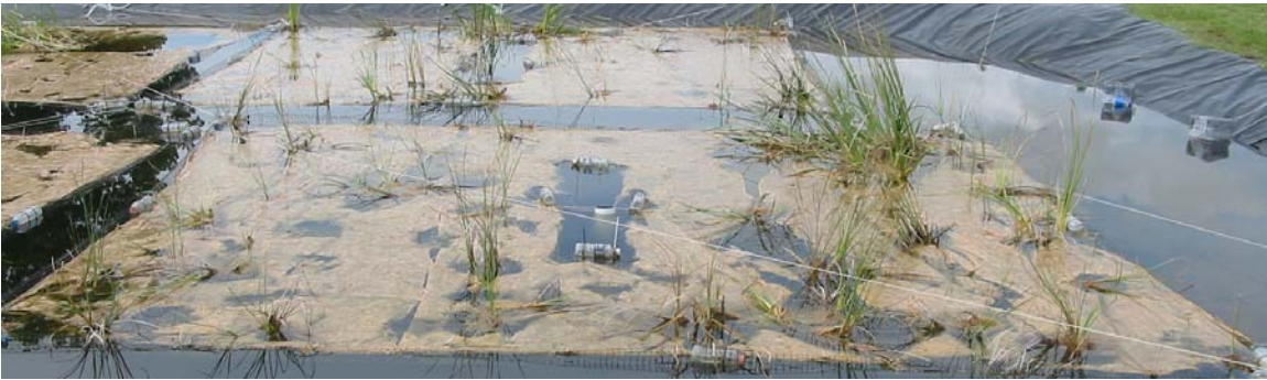
Figure 6.3 EFVM “E” approximately one year after construction and installation
