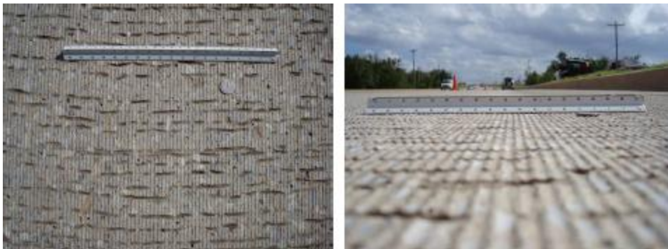
Figure 1.23 Test Section #19 – Diamond Grinding
