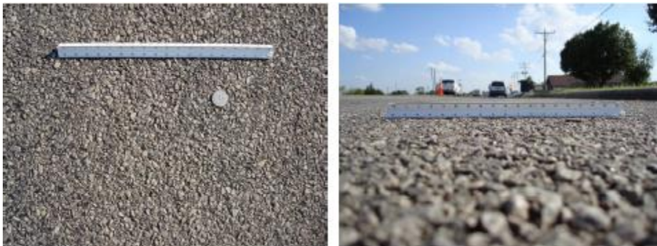
Figure 1.14 Test Section #10 – Chip Seal (3/8'')
