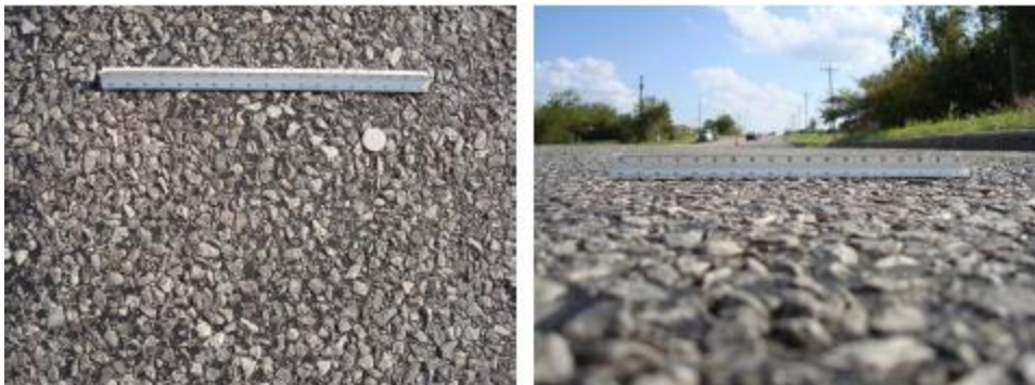
Figure 1.13 Test Section #9 – Chip Seal (5/8'')
