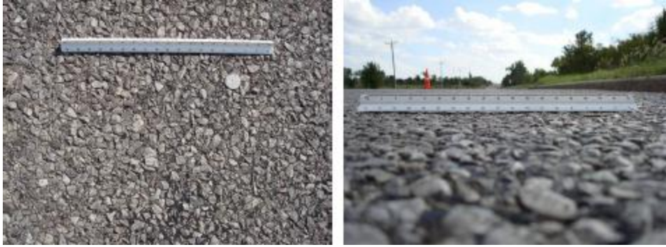
Figure 1.12 Test Section #8 – Chip Seal (5/8'') w/ Fog Seal
