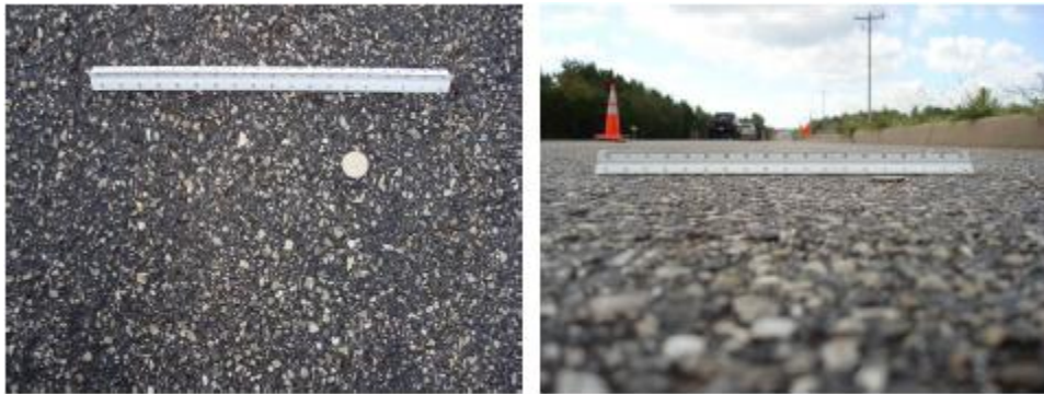
Figure 1.5 Test Section #1 –Calupave Seal
