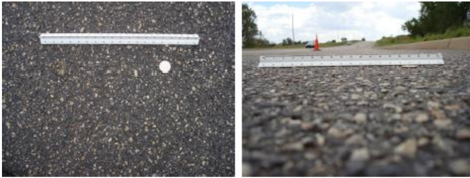
Figure 1.10 Test Section #6 – Asphalt Penetrating Conditioner
