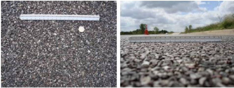
Figure 1.6 Test Section #2 – Open Graded Friction Course w/ Fog Seal
