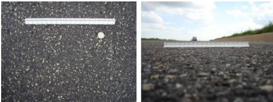
Figure 1.11 Test Section #7 – Asphalt Planer w/ Asphalt Penetrating Conditioner
