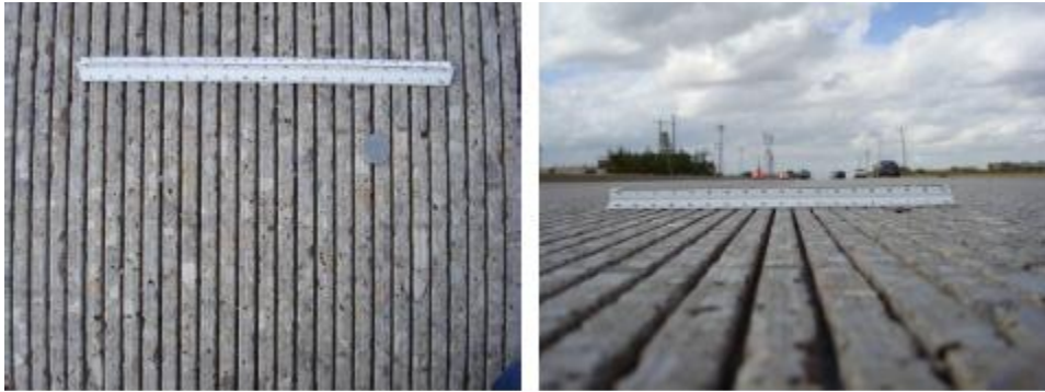
Figure 1.22 Test Section #18 – Next Generation Diamond Grinding
