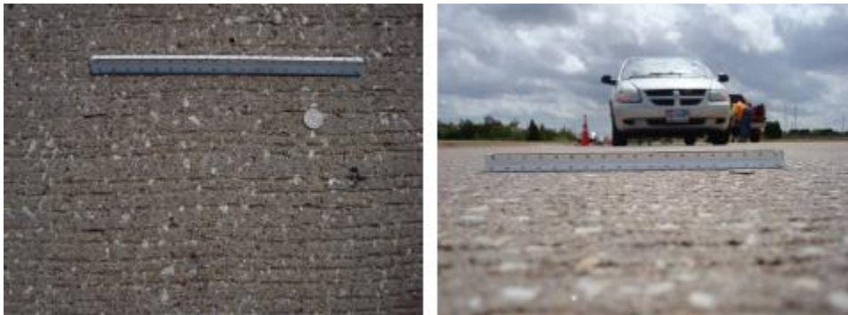
Figure 1.21 Test Section #17 – Shotblasting (Blastrac) w/ Densifier
