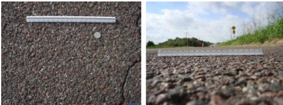
Figure 1.17 Test Section #13 – Shotblasting (Skidabrader)
