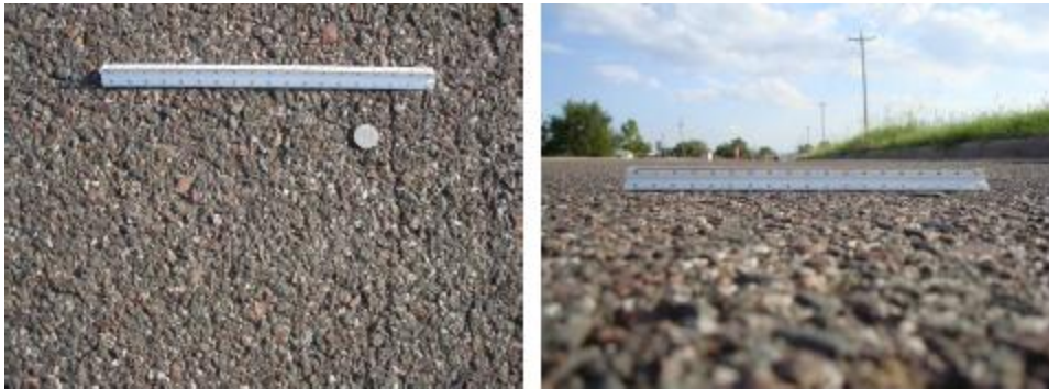
Figure 1.15 Test Section #11 – Shotblasting (Blastrac)
