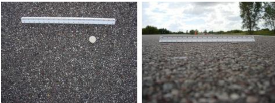
Figure 1.8 Test Section #4 – 1" Mill and Inlay
