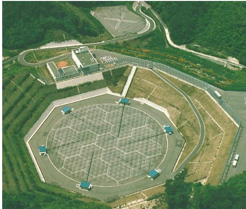
Figure 1.11: Middle and Upper atmospheric radar ( www-lab26.kuee.kyoto-u.ac.jp ). Located in Kyoto, Japan, the device shown is considered one of the most advanced wind profilers of its kind with a received antenna that consists of 475 Yagi elements. The radar is used to investigate atmospheric phenomena and plasma dynamics that occur at high altitudes.
